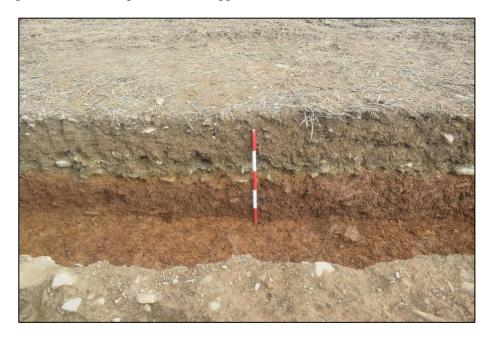
Fig. 7 South-west facing section showing the road construction Photo CPAT 4963-033
