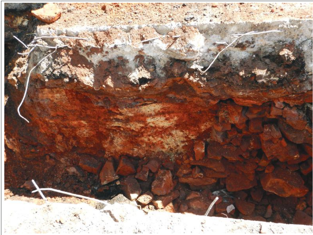
Plate 3. Rubble core of wall [117] visible in base of trench. View to the south. Plate 4. Wall [120] showing stone core of the structure. South facing section.
