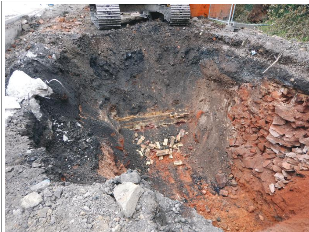
Plate 7. Area 3C. Brick surface [308]. View along the trench to the east.
