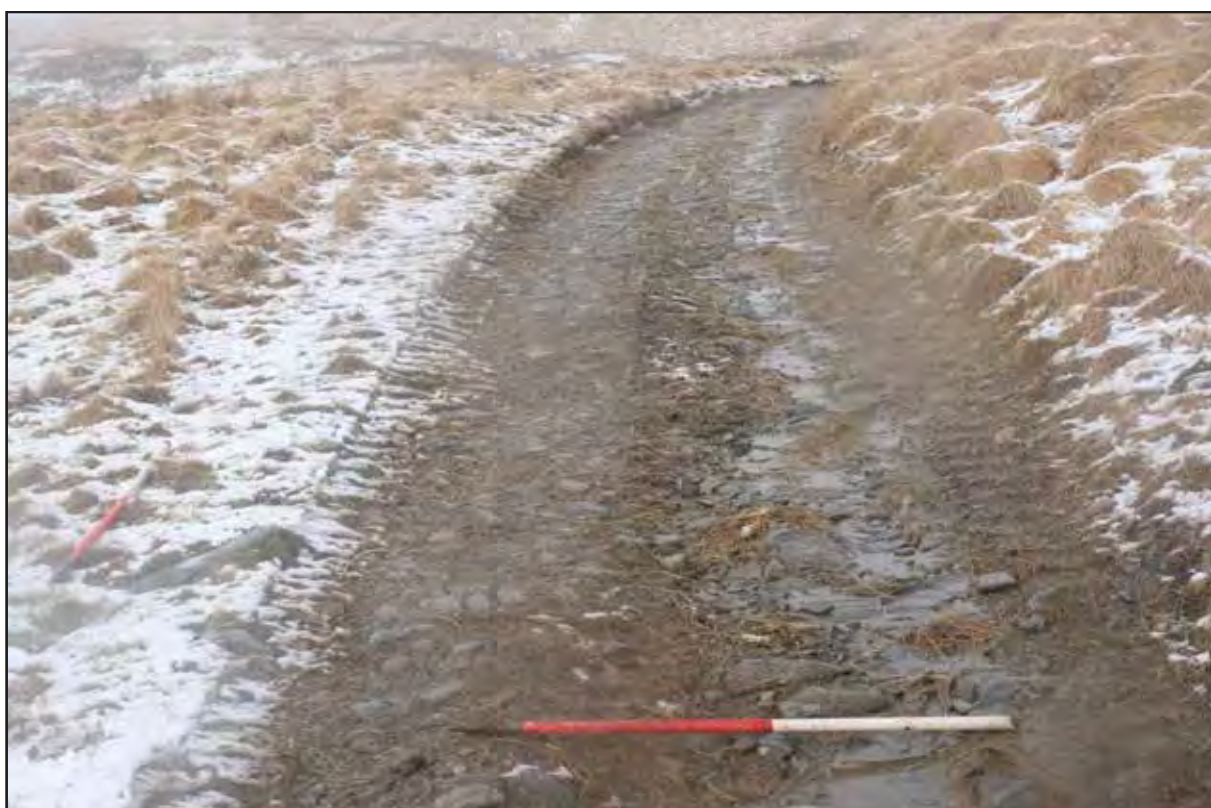
Plate 32 Paved/cobbled surface and kerbstones, found to the immediate west of area 8 (western area of scheme)
