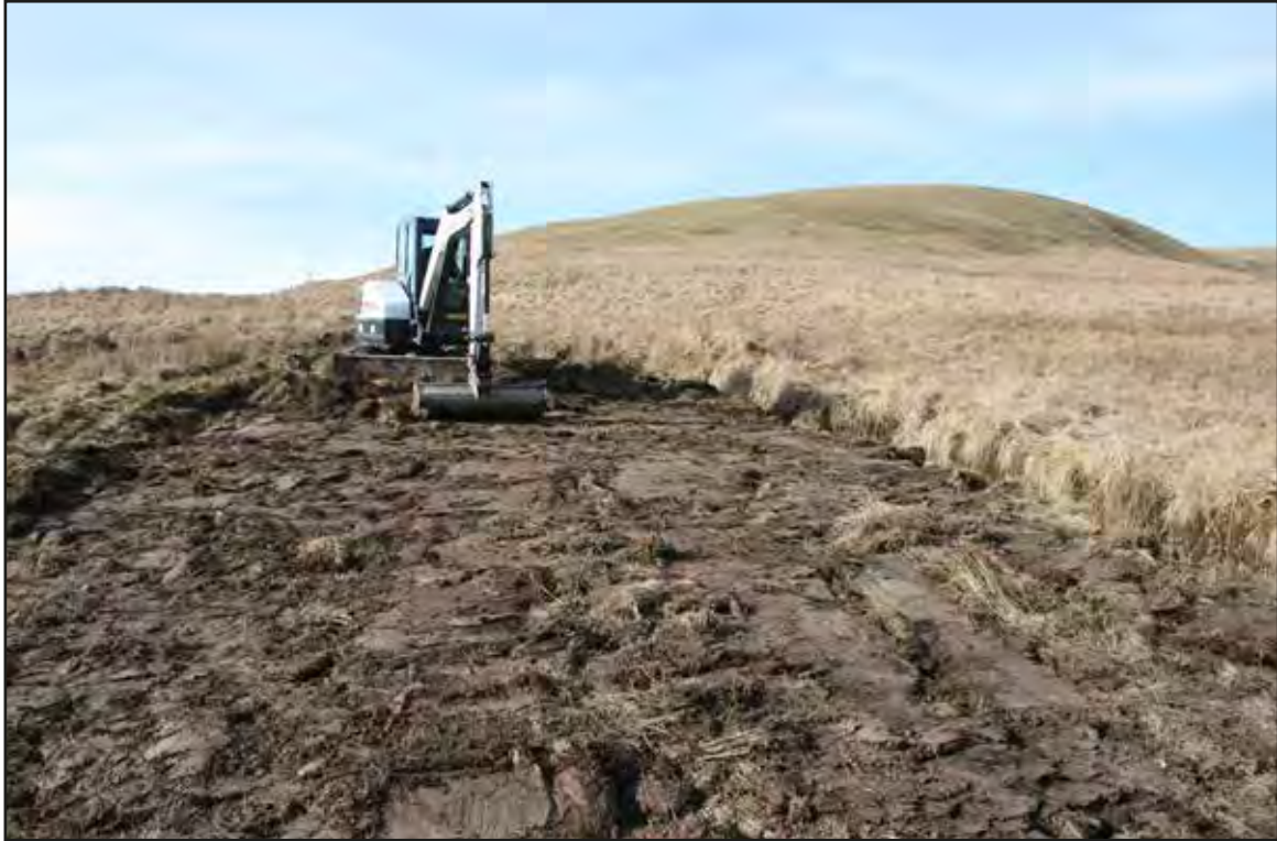
Plate 1 Work being conducted in area 1 (east end of scheme). View south-west.
