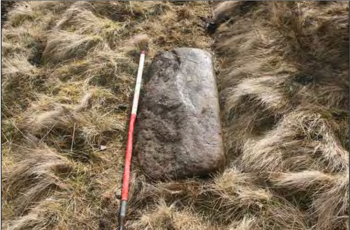
Plate 21 Displaced kerb stone found during area 1 works (western area of scheme)
