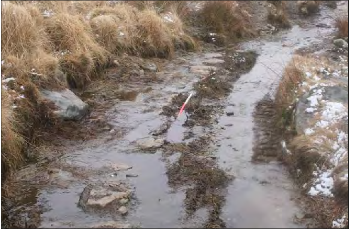
Plate 29 Paved surface and kerbstones, found to the immediate west of area 7 (western area of scheme)
