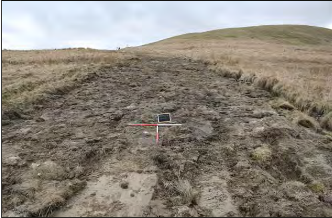
Plate 3 View south-west of work completed within area 1 (eastern area of scheme)
