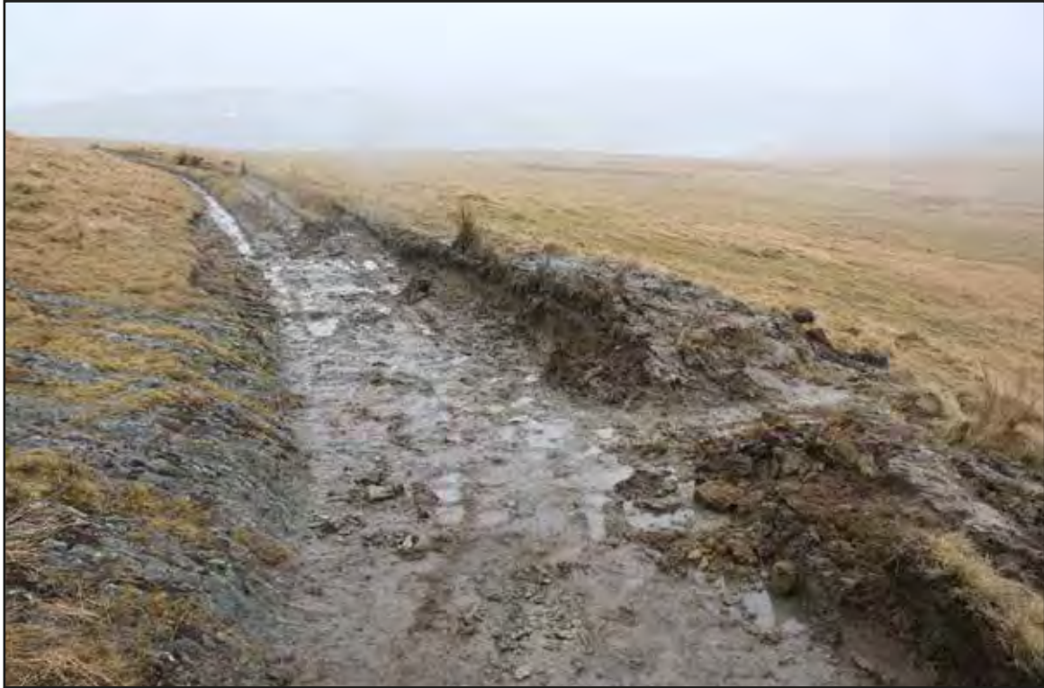
Plate 7 View east of drainage grip installed within area 4a (eastern area of scheme)
