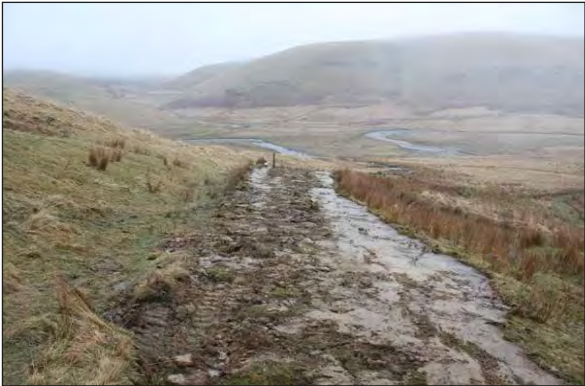
Plate 6 View north-east of groundworks completed within area 3 (eastern area of scheme)
