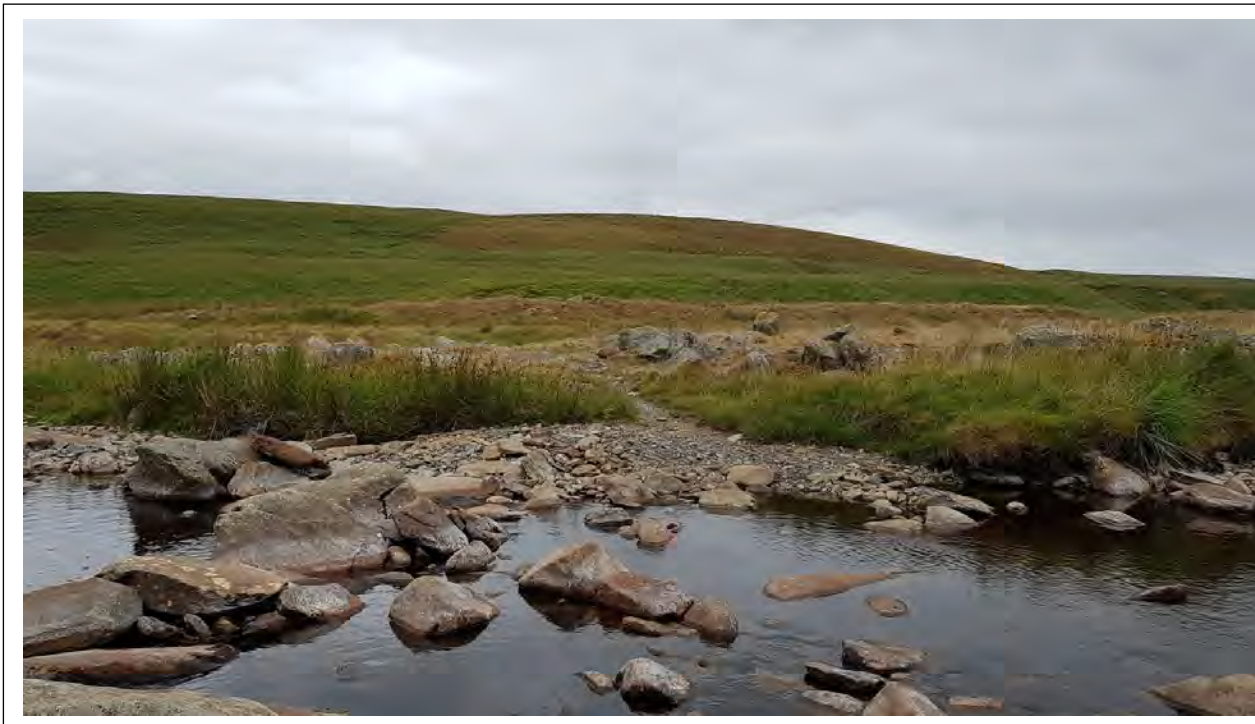
Plate 75. View of Monks Trod trackway, looking southwest at ford on Avon Claerwen NPRN 67752
