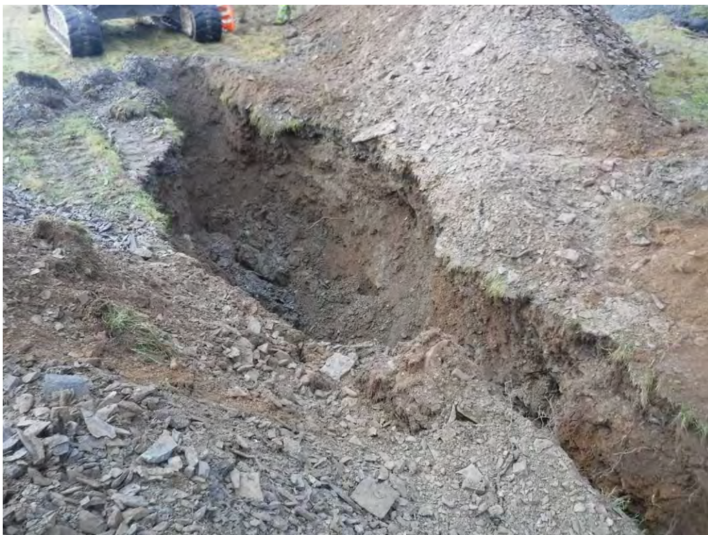
Photo 40. Trial Trench/TP112, facing west, showing deposits 11204, 11203, 11202, 11201 & 11200.
