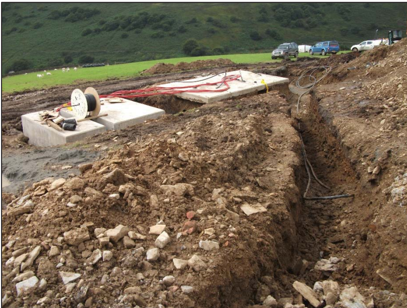
Plate 2: Transformer bases
