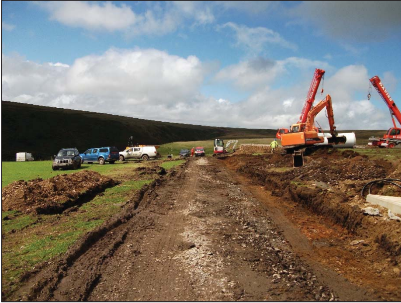
Plate 1: Access road between turbine bases.
