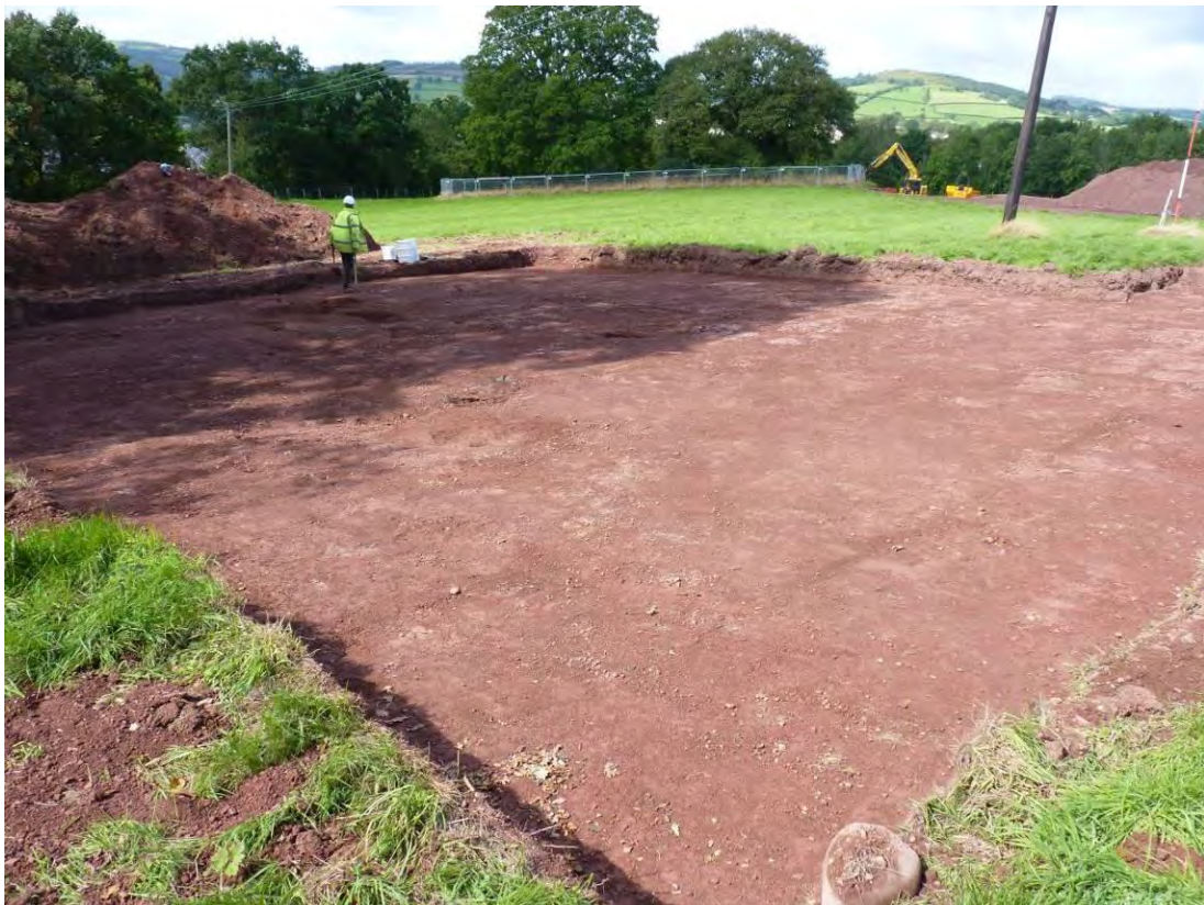
Photo 2: General shot looking west across the excavated area.
