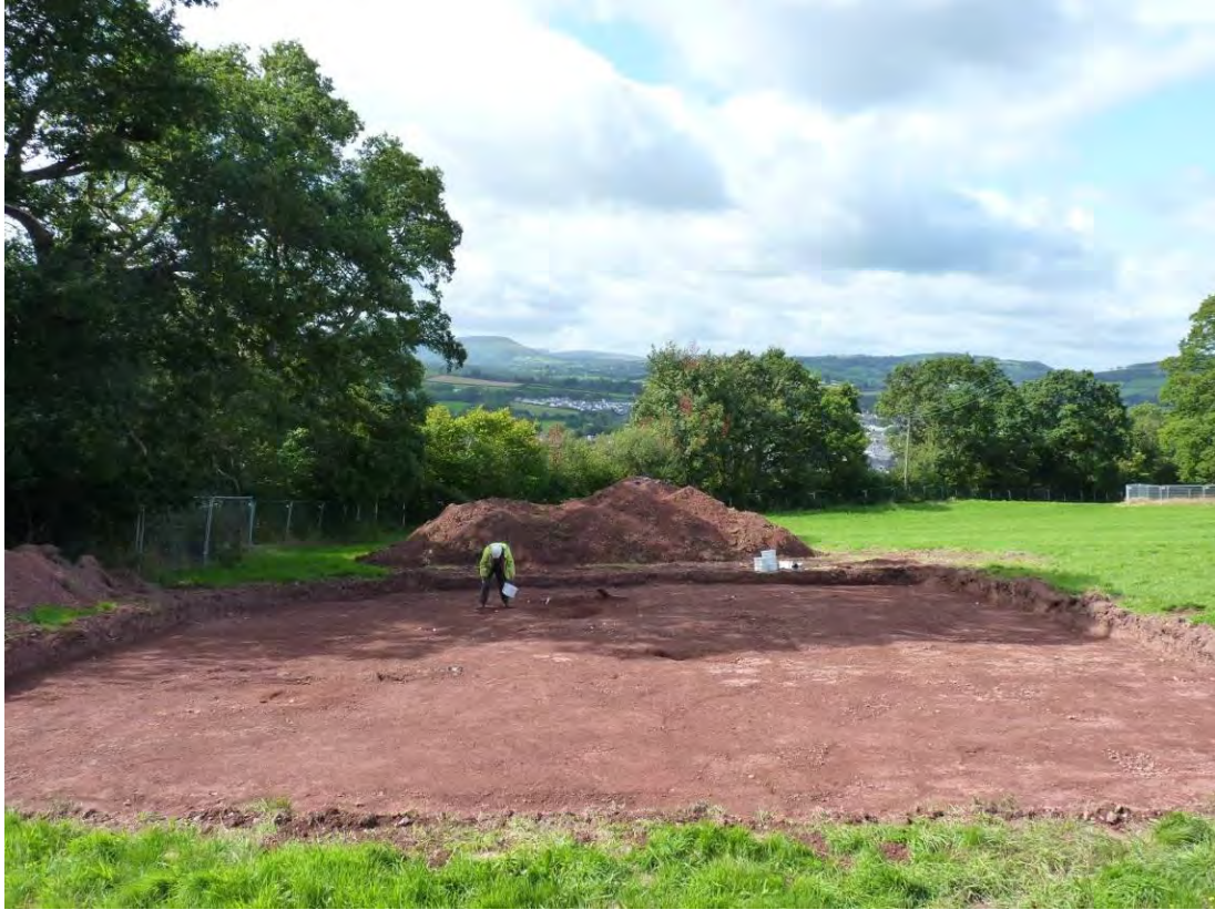
Photo 1: General shot looking southwest across the excavated area.
