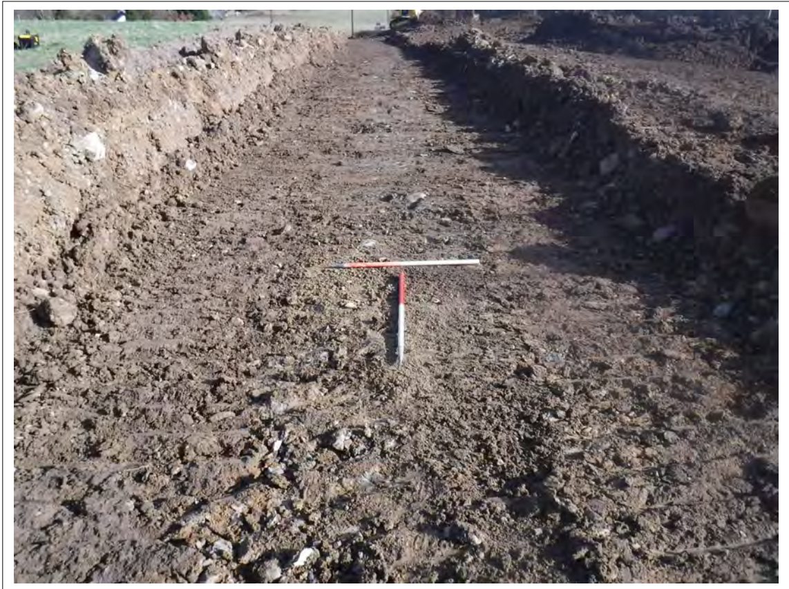
Plate 1. Area A after strip looking north. Scales 2 x 1m
