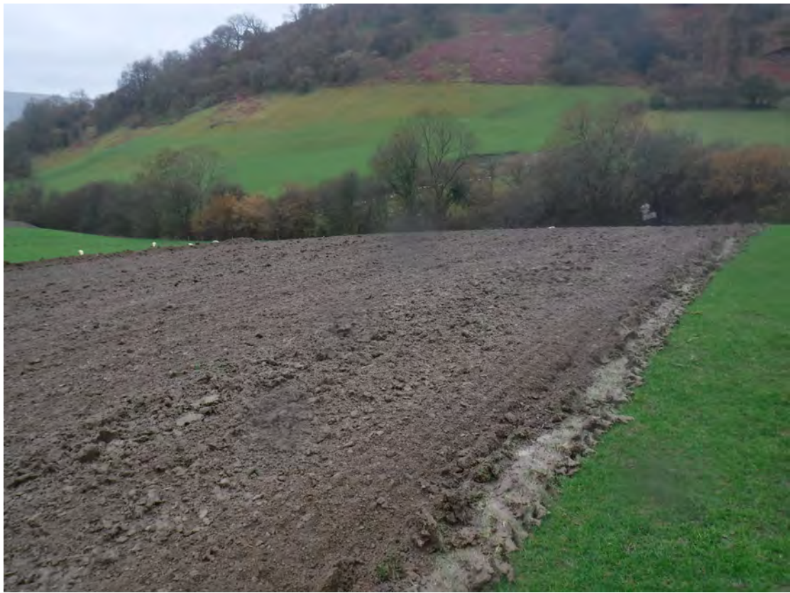
Plate 5. Working shot, stripping topsoil (2001) within Area B, looking southwest.
