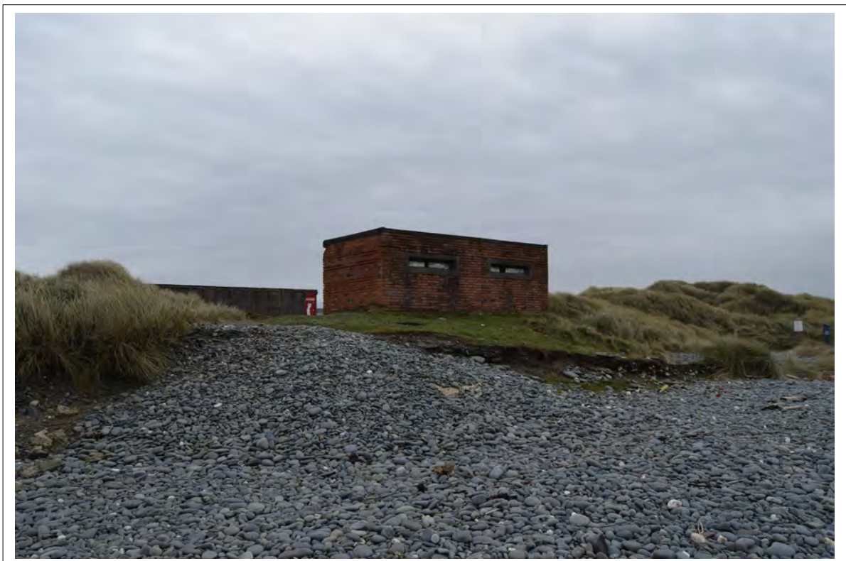
Plate 2. Military building, looking SE
