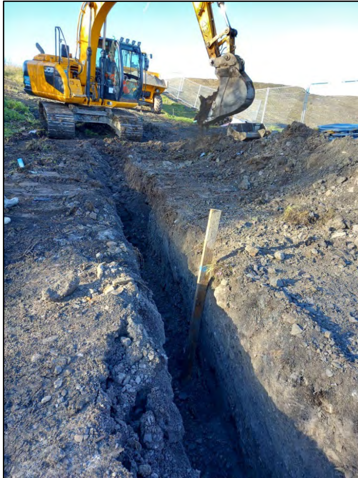
Plate 1: Excavation of Cable Trench, Working shot, View to NW
