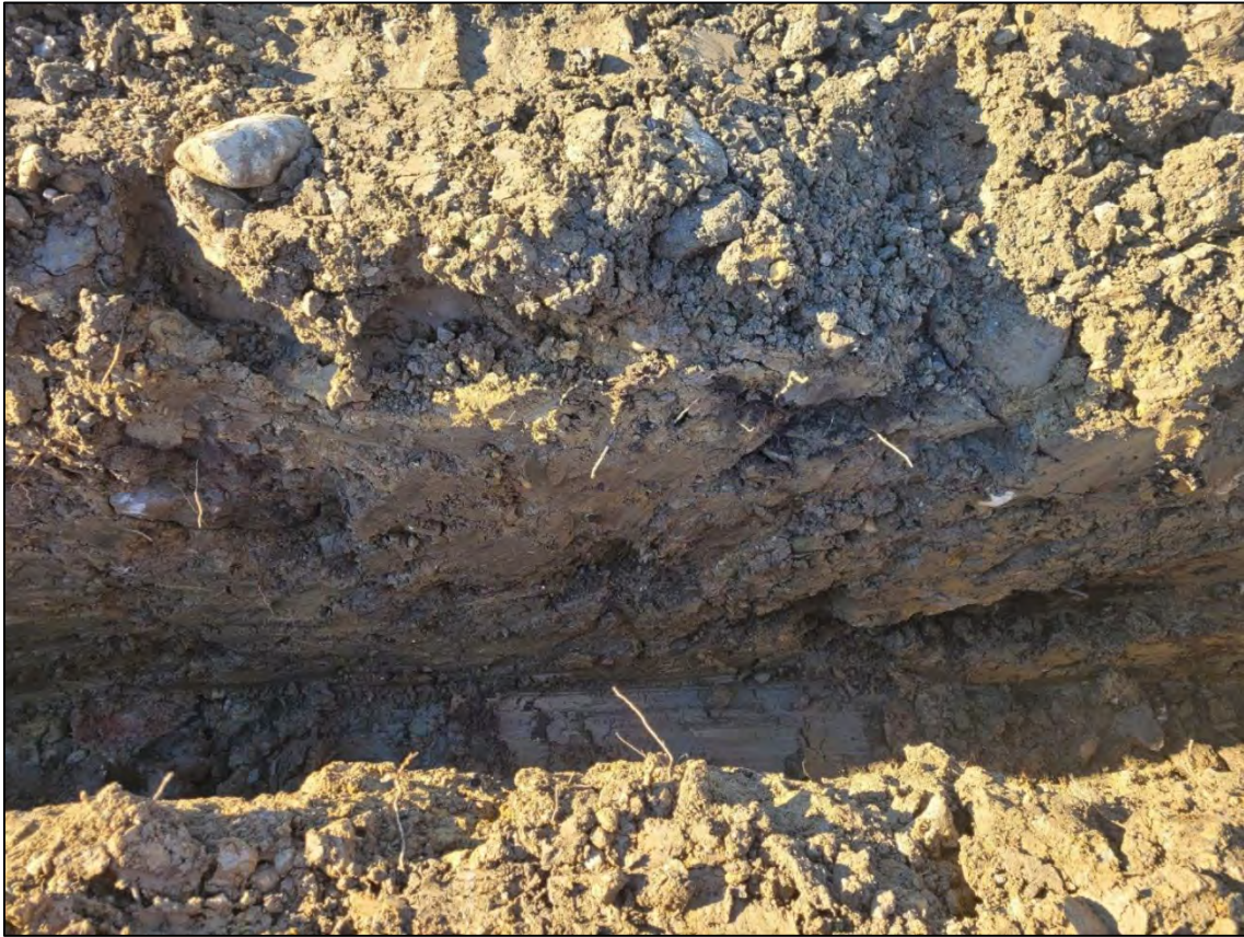
Plate 5: Cable Trench N of A465, E facing Section, View to W
