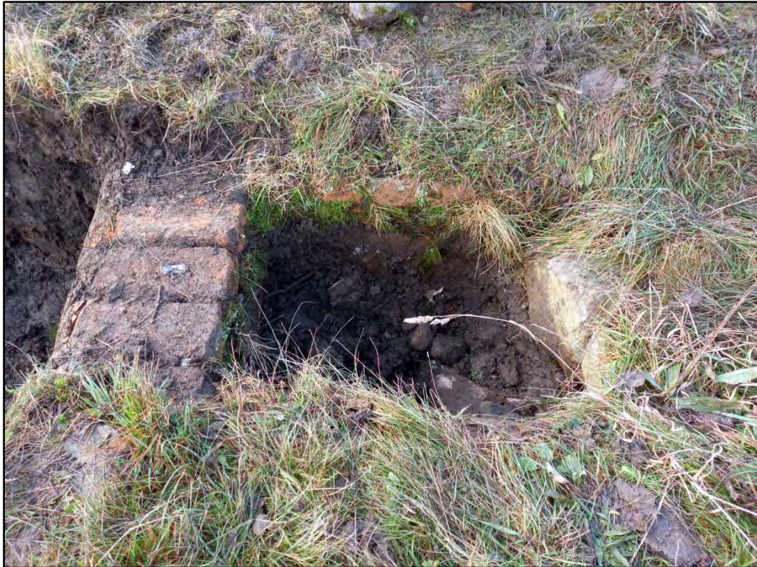
Plate 3: Manhole (103), View to NW
