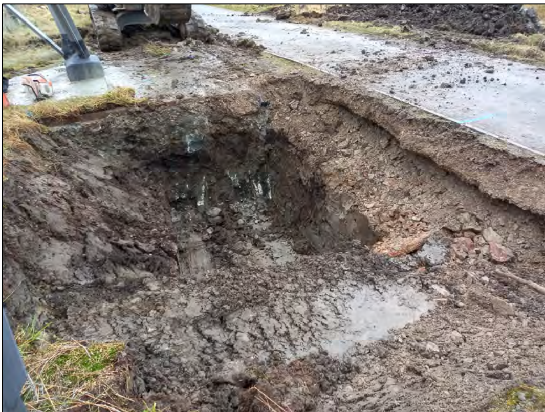
Plate 8: DD3A Test Pit 1, SW of existing pylon, View to SE
