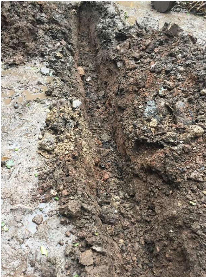
Plate 6. Excavation of drainage trench, north-east facing
