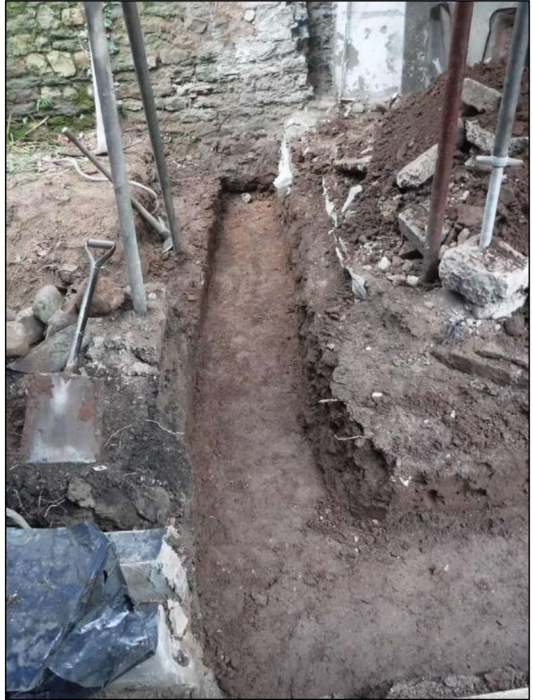
Plate 1. North-west to south-east area of foundation trench
