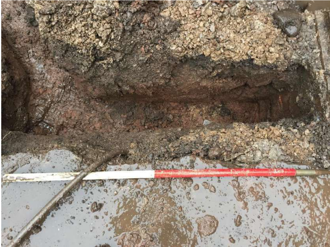
Plate 7. Excavation of drainage trench, south facing – 1m scale
