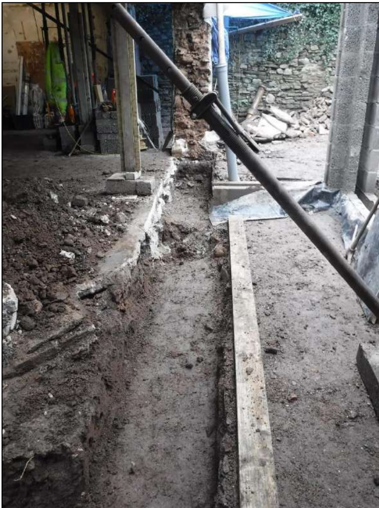
Plate 2. South-west to north-east area of foundation trench
