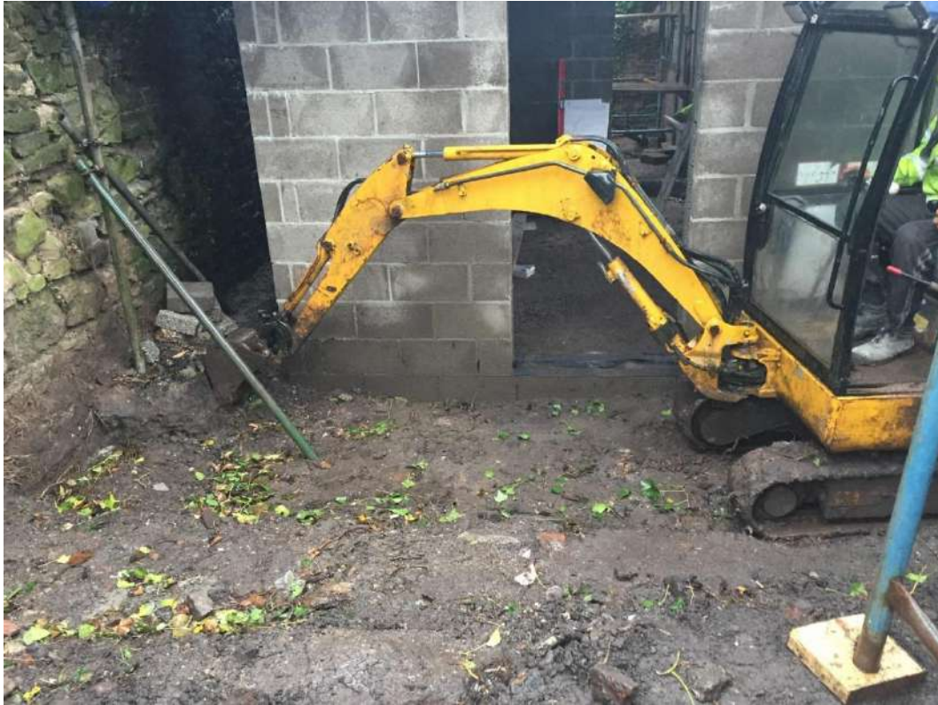
Plate 3. Excavation of drainage trench – north-west facing
