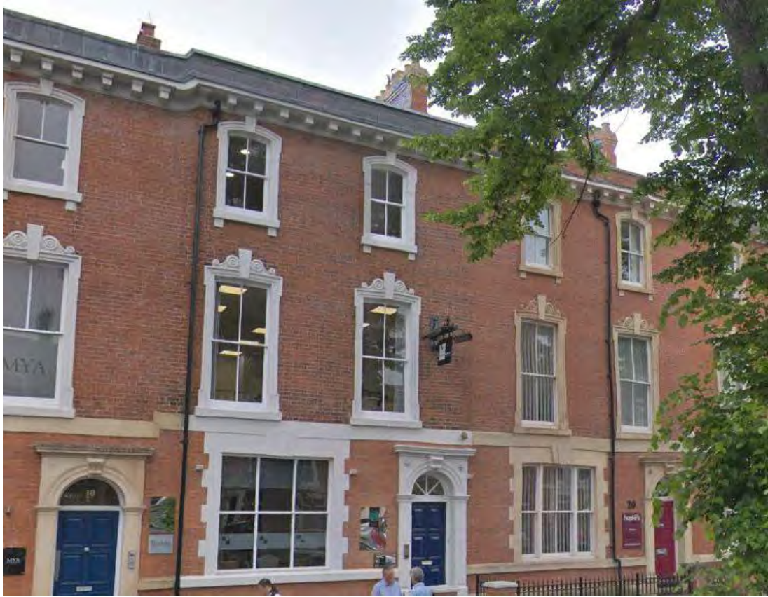
Photo 1: The frontage of No.19 Windsor Place, as viewed from Windsor Place.
