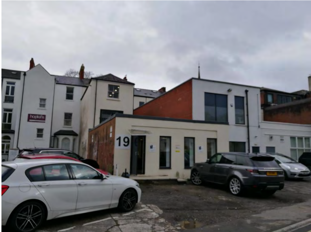
Photo 5: More detailed view of the rear extensions to No.19 Windsor Place.
