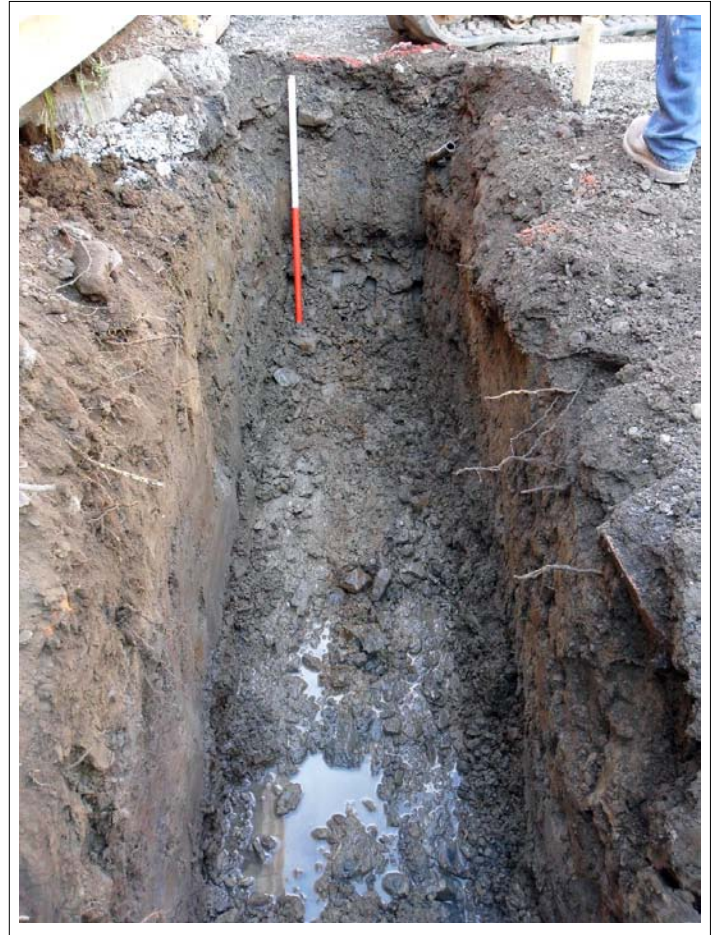
Plate 4: View along southern foundation trench looking west, Scale 1x1m
