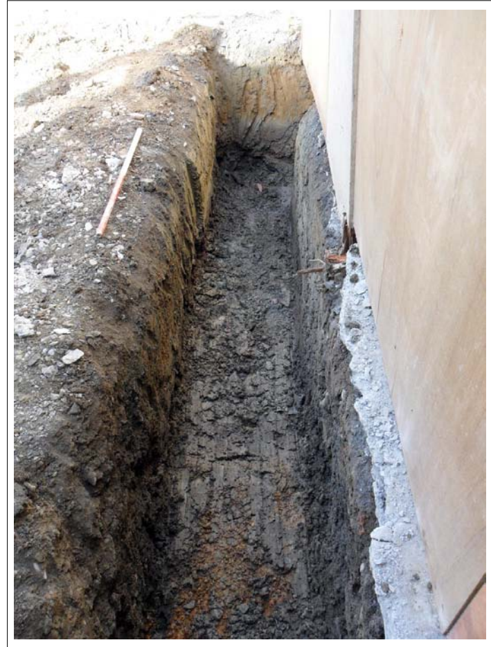
Plate 2: View along northern foundation trench Looking south west, Scale 1x1m
