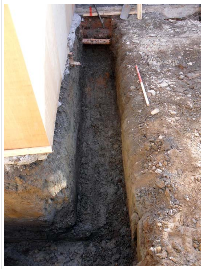
Plate 1: View along northern foundation trench Looking north east, Scale 1x1m
