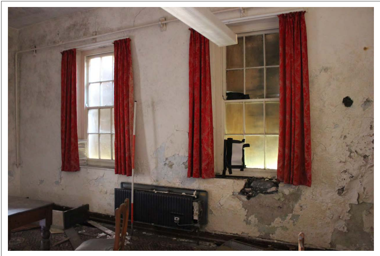
Plate 13: View east showing vestry sash horned windows
