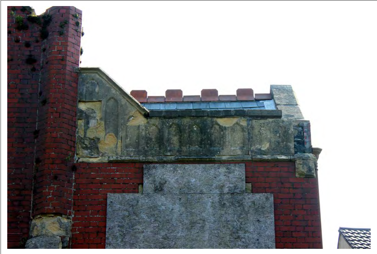
Plate 4: Western elevation parapet with blind lancets
