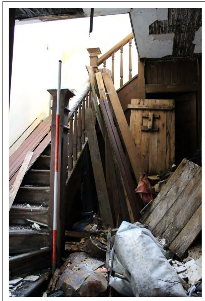
Plate 42: View south showing stairs leading to upper balcony
