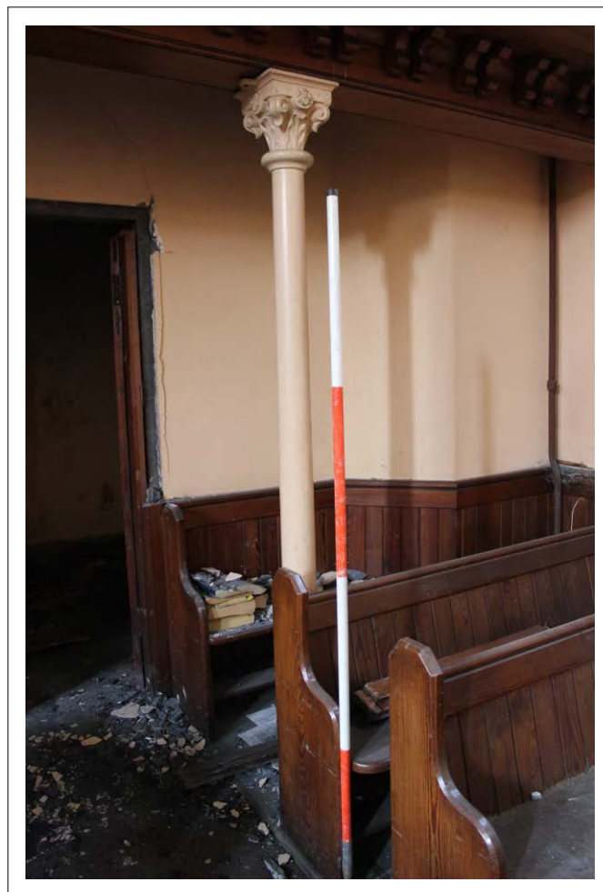
Plate 18: View west showing detail of columns
