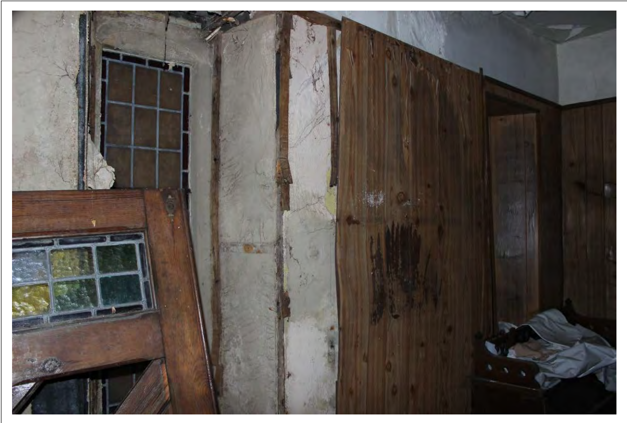
Plate 41: View north west showing windows in side room
