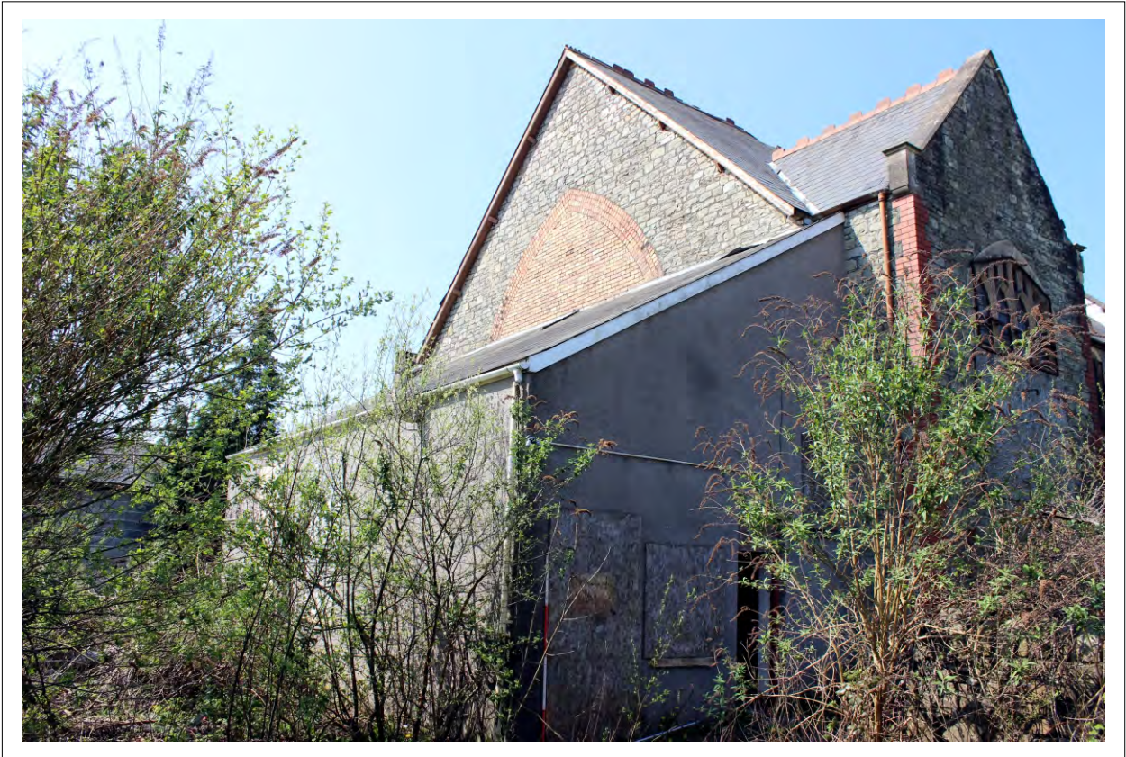
Plate 9: Eastern elevation pent roofed vestry
