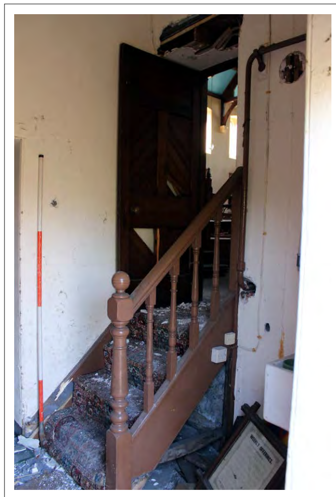
Plate 10: View from vestry doorway, south toward stairs leading into chapel
