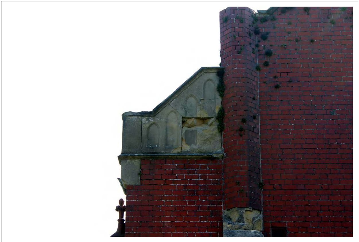
Plate 3: Western elevation parapet with blind lancets
