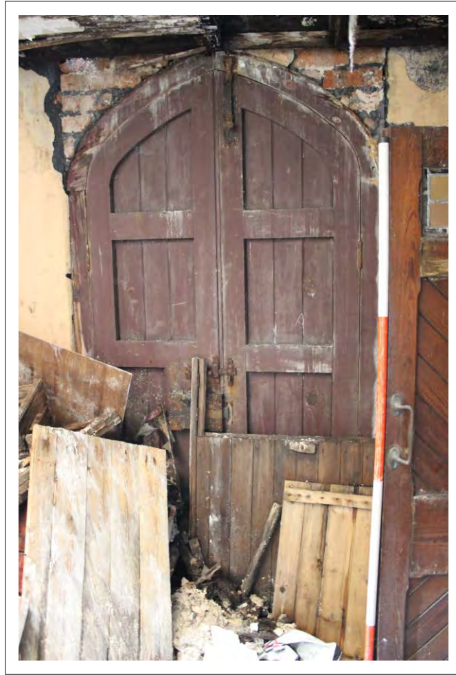
Plate 43: View west showing side doorway
