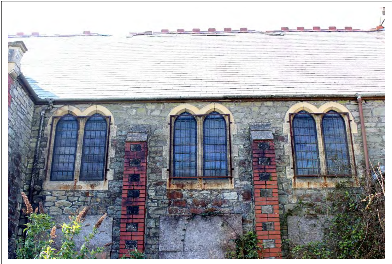
Plate 7: Northern elevation upper windows
