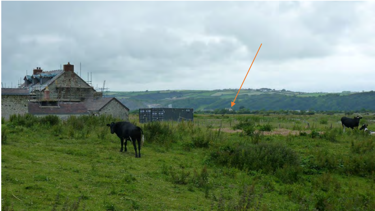
Photo 7: View NW from adjacent to East House, a similar characteristic Georgian style farmstead incorporating Listed Buildings, demonstrating poor visibility with intervening vegetation cover. Arrow points to Hurst House.
