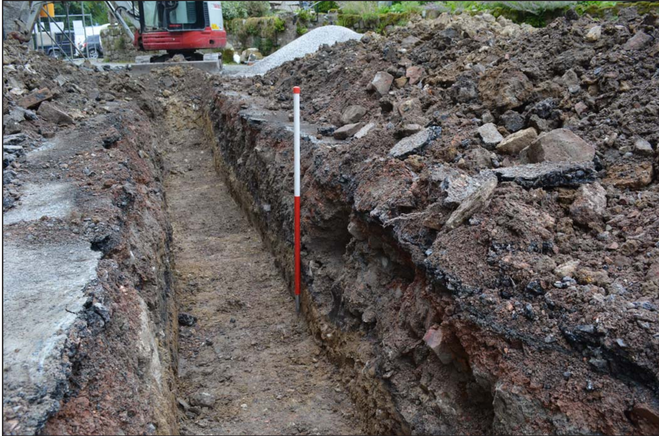
Plate 15: Main drain trench, from the north. Scale 1.0m.
