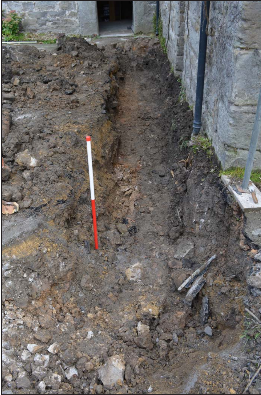
Plate 11: Drainage connection C3, from the southwest. Scale 1.0m.
