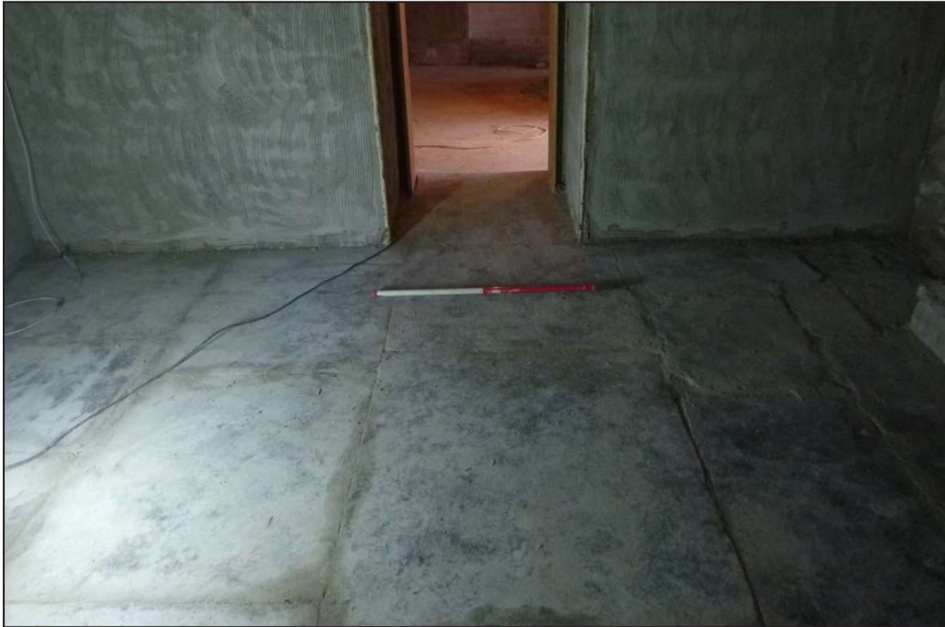
Plate 20: Lobby (G3) showing existing flagged floor, from the southwest. Scale 1.0m.
