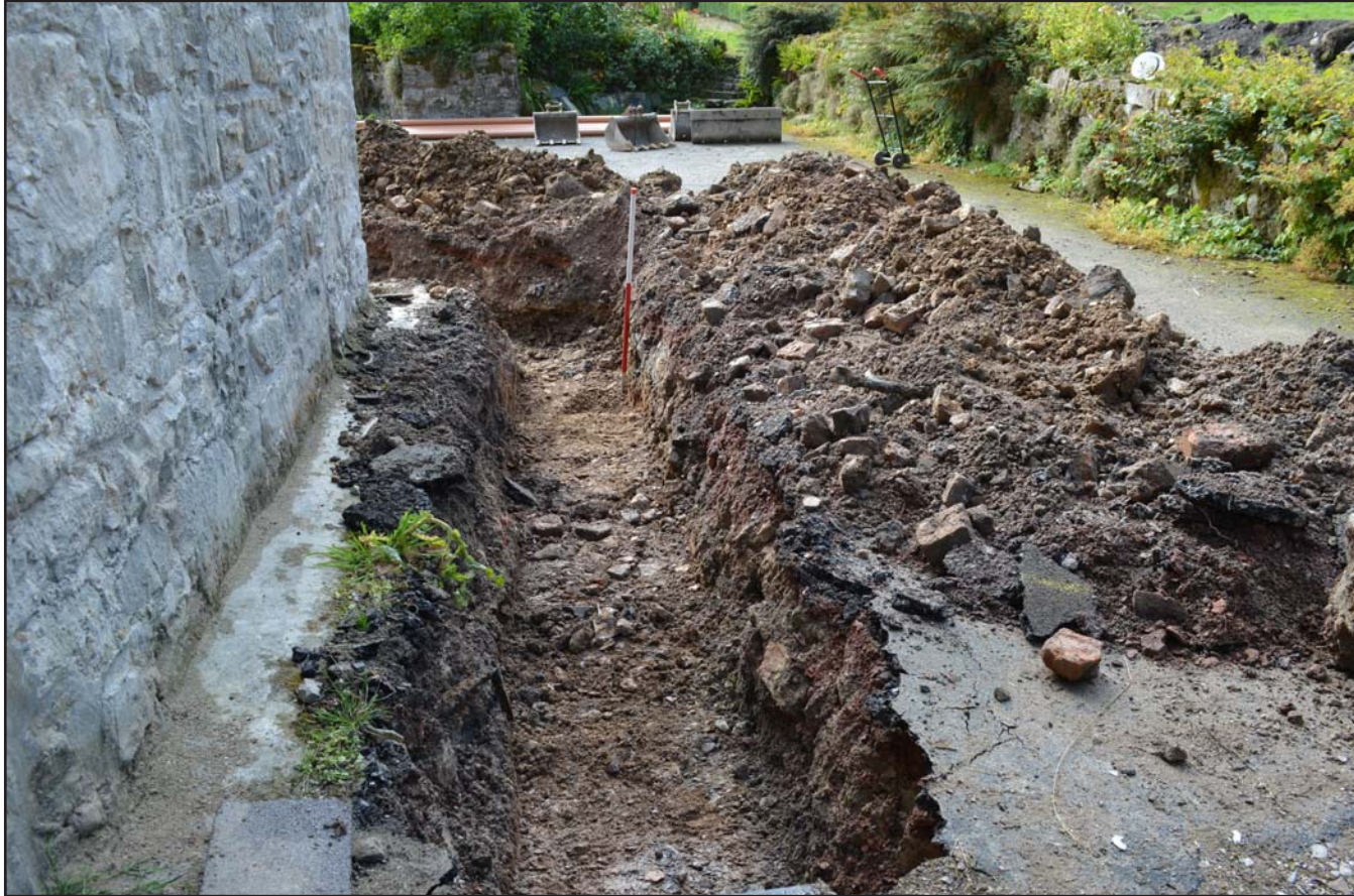
Plate 03: Main drainage connection, from the northeast. Scale 1.0m.
