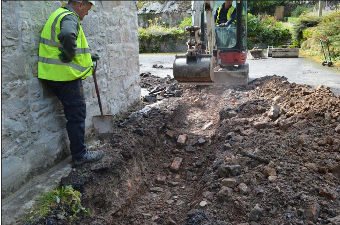
Plate 02: Excavation of main drainage connection, from the northeast.
