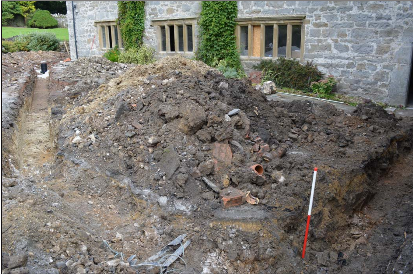
Plate 17: General shot showing drainage trenches, from the southwest. Scale 1.0m.
