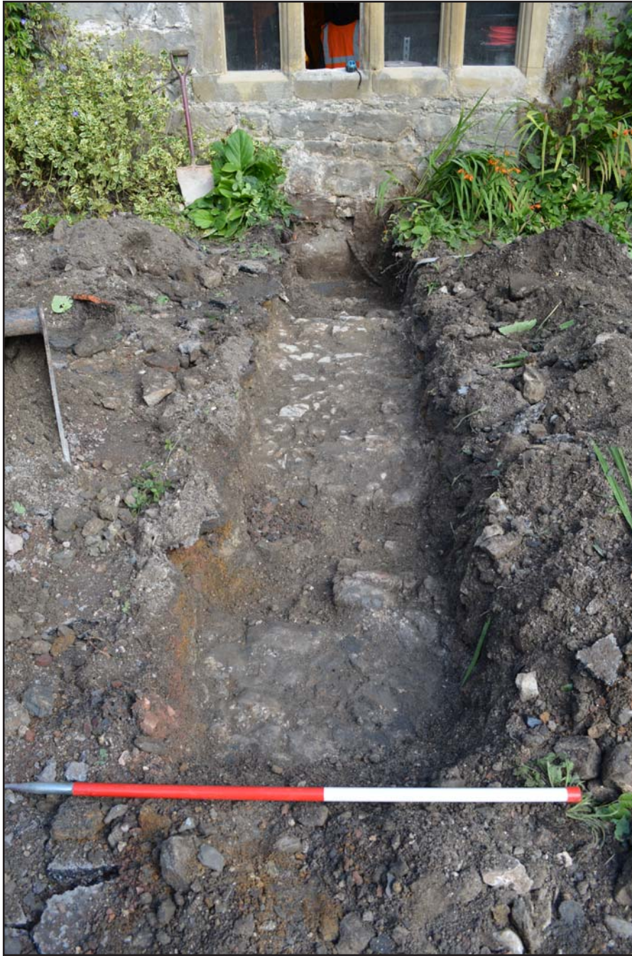
Plate 07: Drainage connection C1 showing cobble deposit (08), from the southwest. Scale 1.0m.
