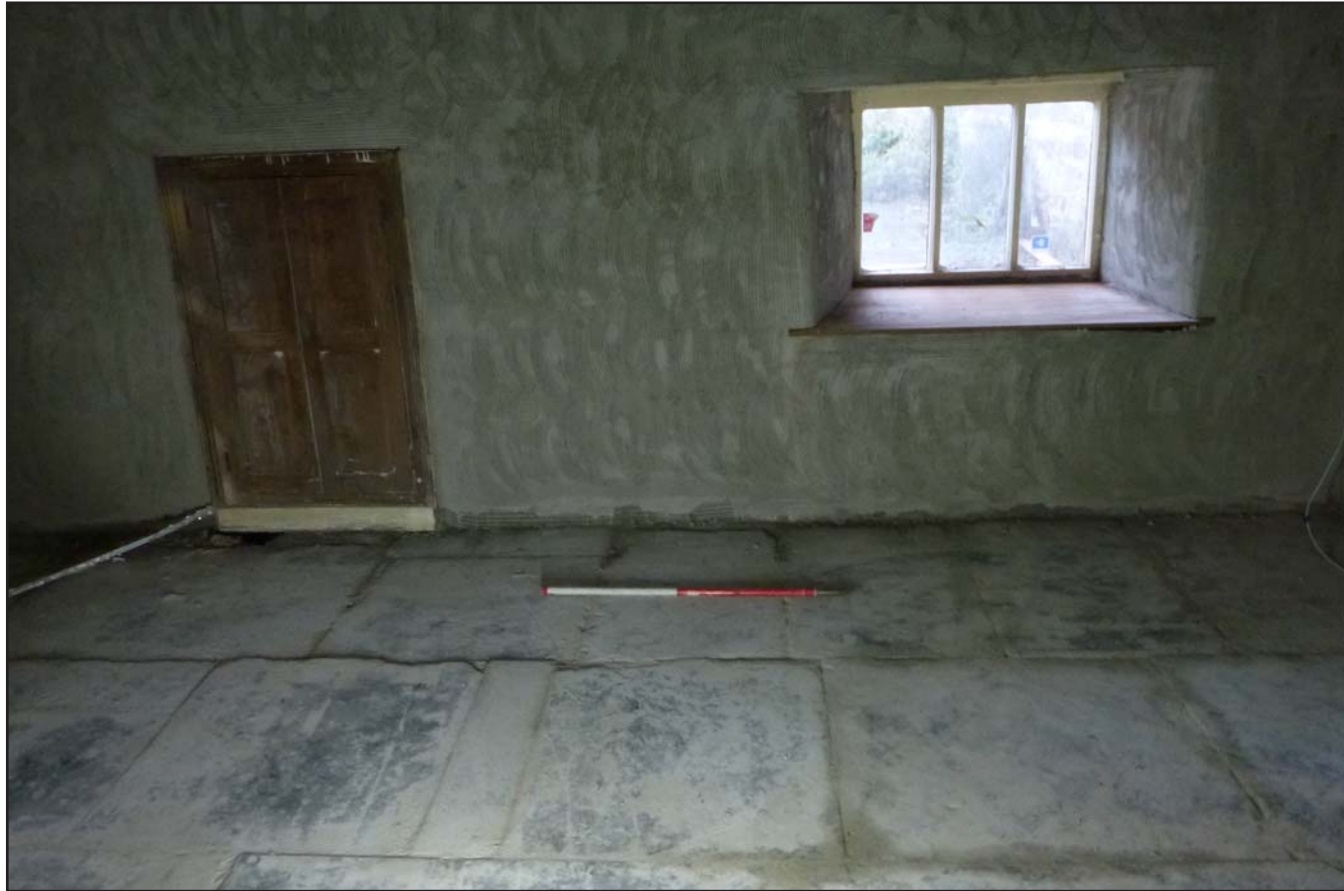
Plate 21: Lobby (G3) showing existing flagged floor, from the southeast. Scale 1.0m.
