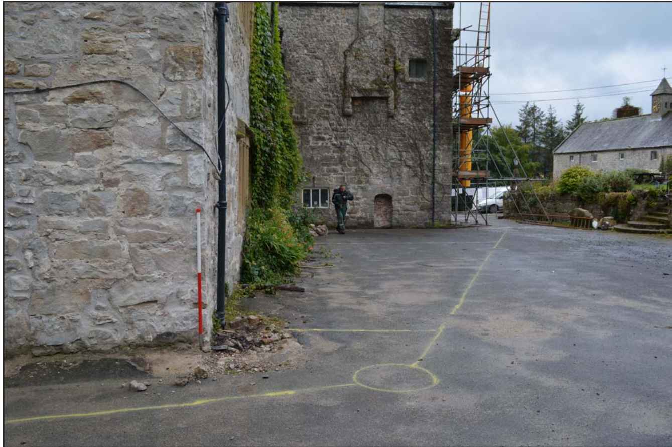
Plate 12: Pre excavation main drain location, from the north.
