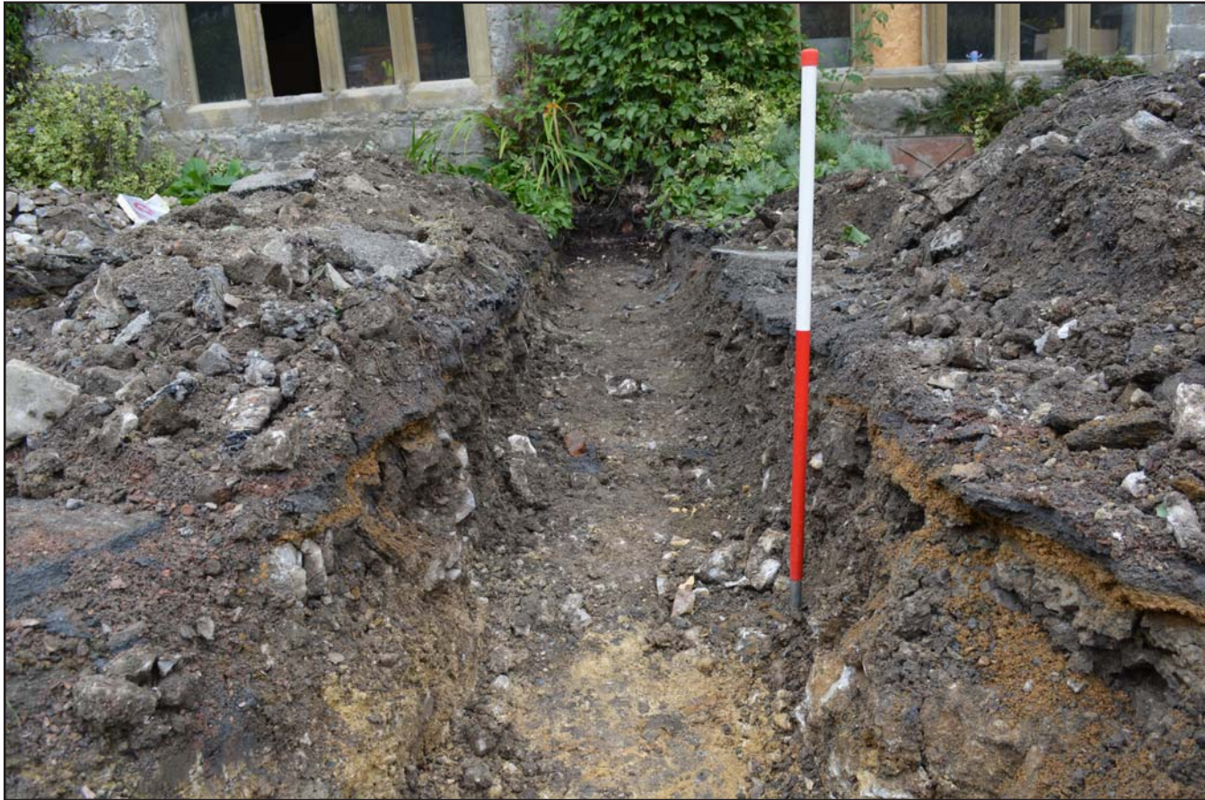
Plate 10: Drainage connection C2, from the southwest. Scale 1.0m.
