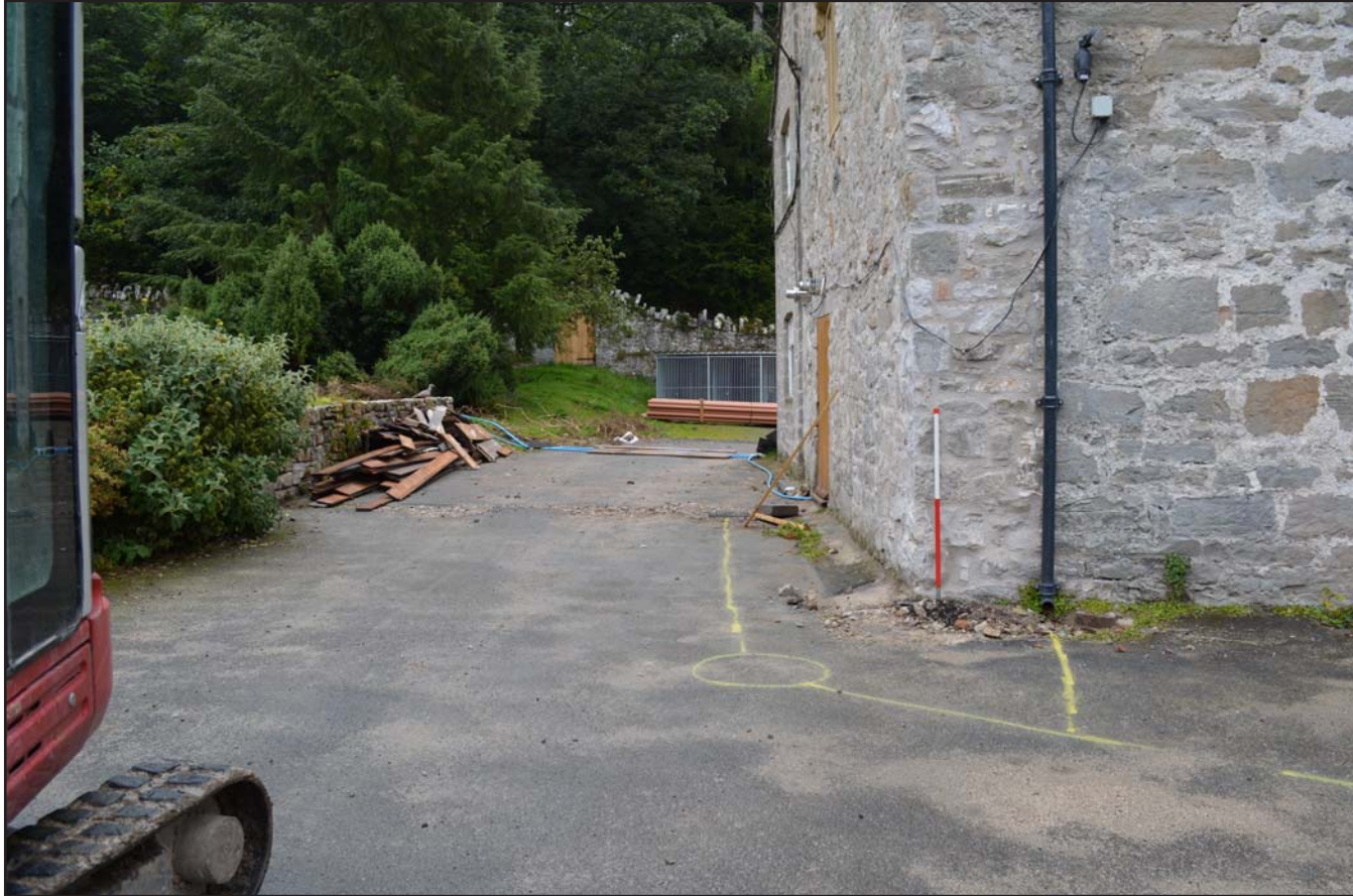
Plate 01: Pre excavation main drainage connection, from the southwest. Scale 1.0m.
