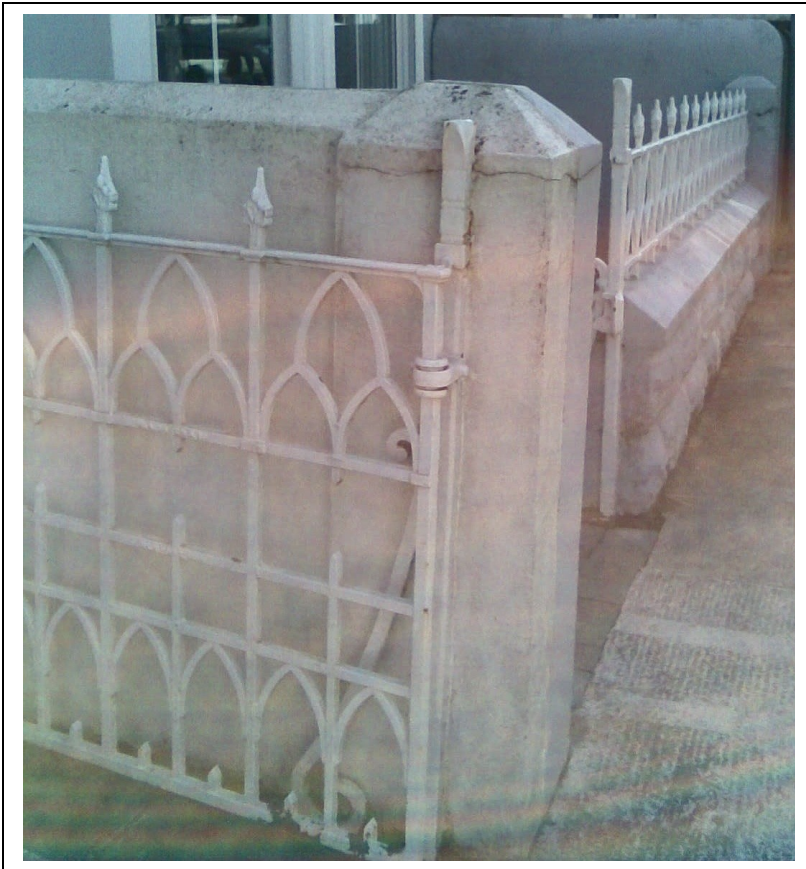
Elmbrae (front railings no gate) Haskell Cottage (gate, no railings)
