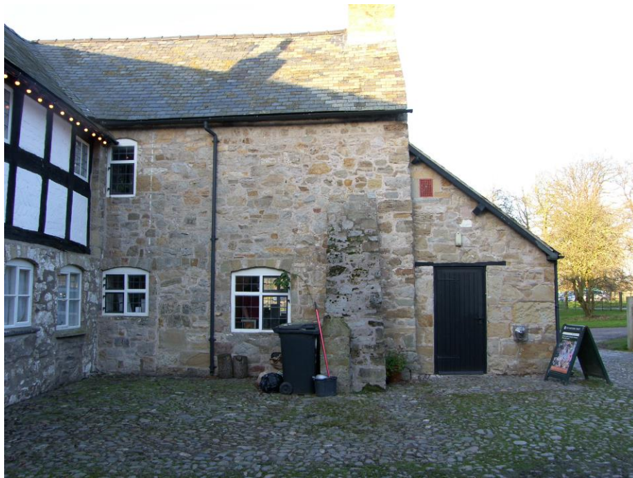
47 Rear of Johnson’s Cottage with part of The Both (left)). Late C16th – early C17th origin. Johnson’s Cottage has been completely modernised internally. PM A . Note the blocked door on left, probably a mid/late C19th change.
