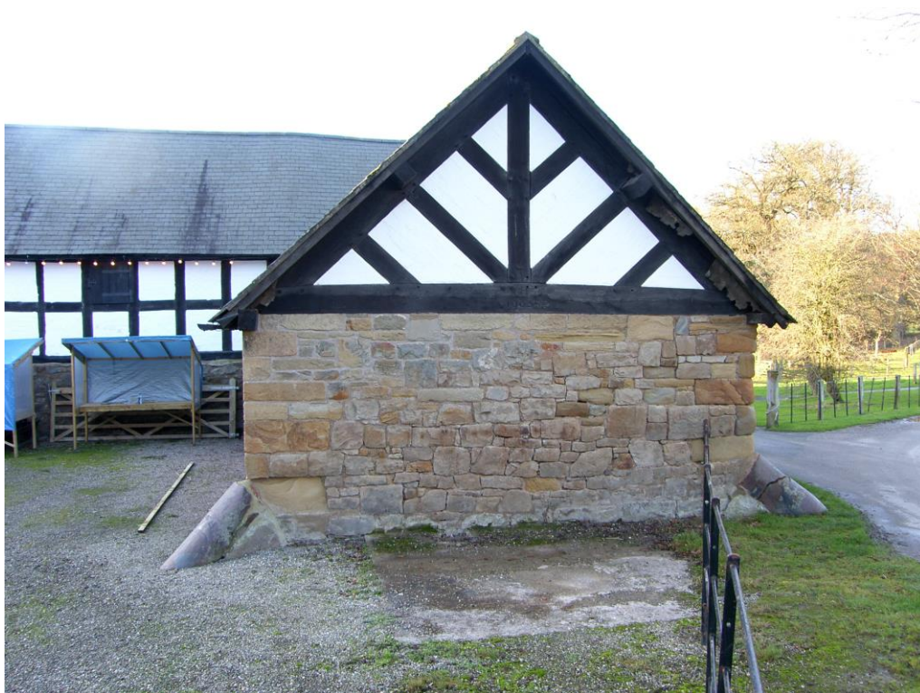
33 Open fronted Cart or Implement Shed – early C20th with feeding trough and cobbled floor. PM K . Note curious cylindrical corner reinforcement – purpose unclear.
