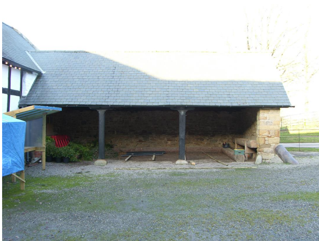
29 Open fronted Cart or Implement Shed – early C20th with feeding trough and cobbled floor. PM K
