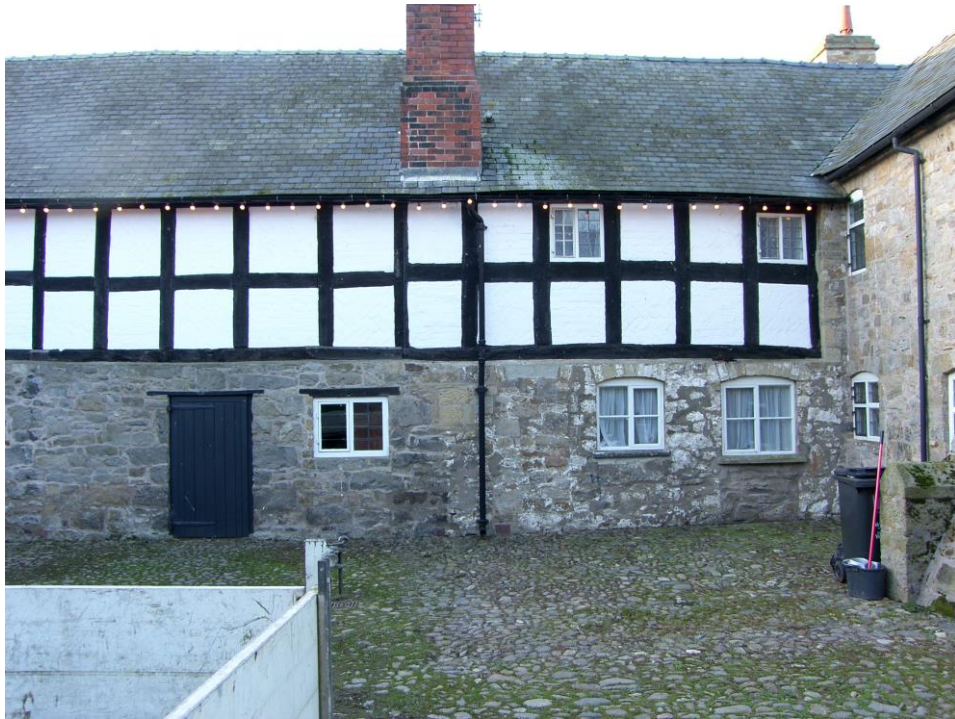
46 Part of the coal-shed (see previous) and the Bothy (right). Note break in masonry between the two. Both early-mid C18th – possible the Bothy was formerly an annexe of Johnson’s cottage before Home Farm complex was built. PM D C
