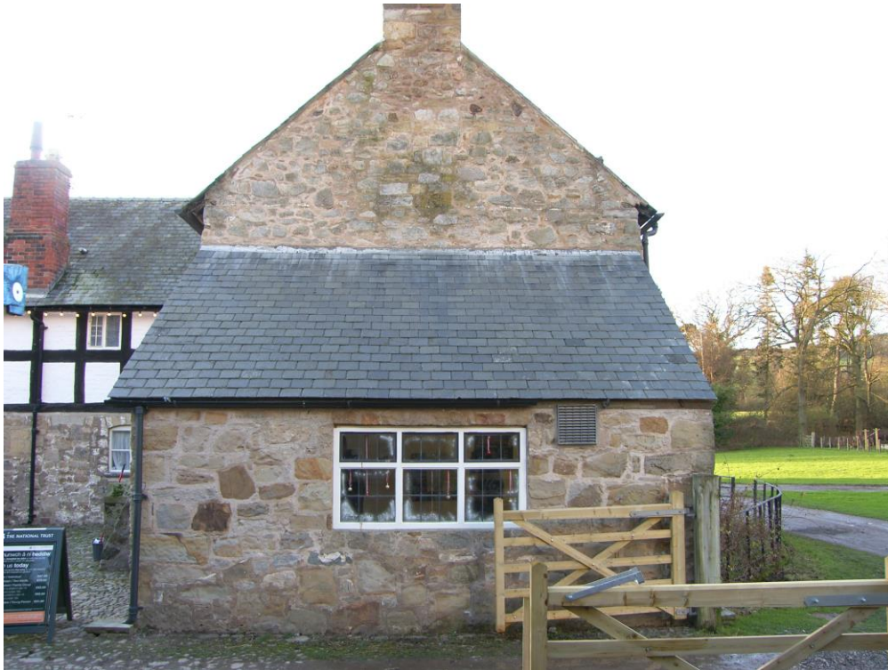
56 Johnson's Cottage, outshot with catslide roof, possibly a late addition, built at time of Open fronted Implement Shed PM K (see view 33 above). Early C20th. PM A
