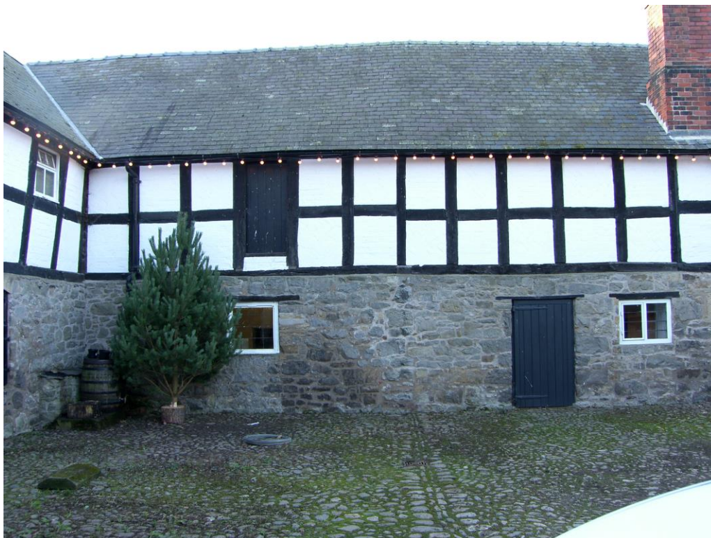
45 Lofted Cowhouse (left), former coal-shed and privy (right). early-mid C18th. PM E D Note blocked door between door and window (C19th modification)
