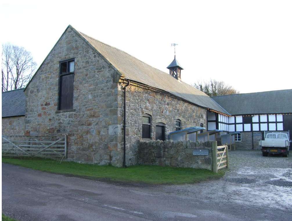
37 Oblique view of Stable, lofted with hay loading eye to upper floor storage area. ?late C18th. PM J I
