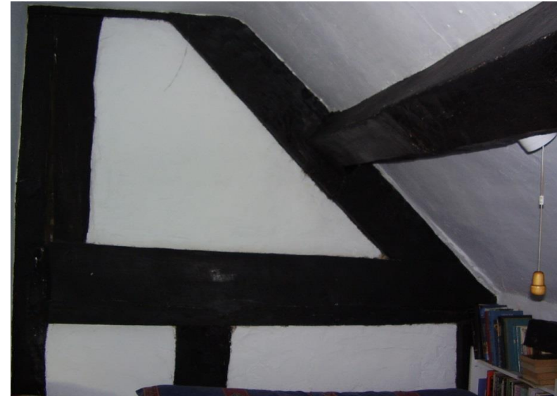
Fig 7. Part of cruick beam in upstairs bedroom.
