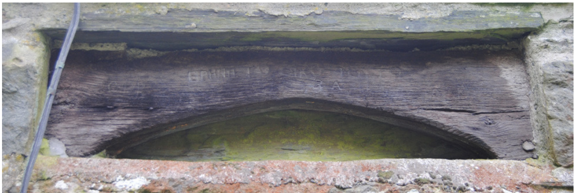
Plate 5: (?)Primary doorhead reset in masonry of west wall above current door
