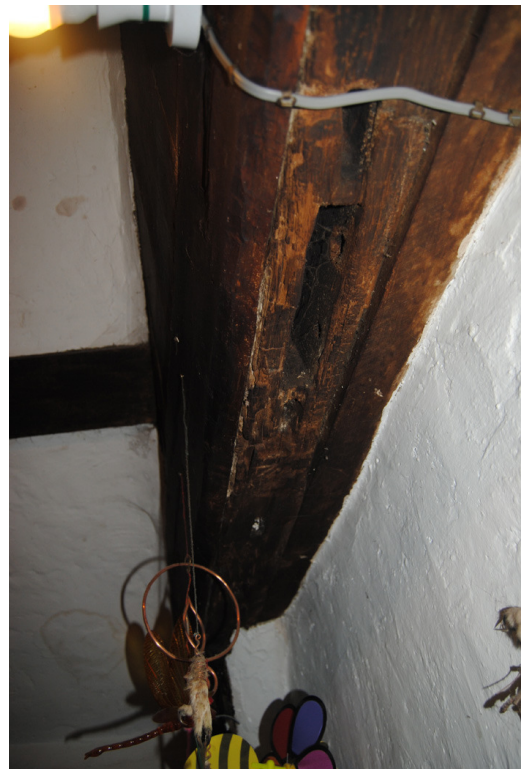
Plate 27: Mortices to collar soffit of C1.
