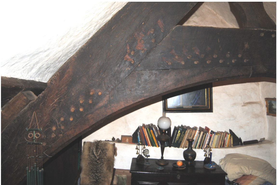
Plate 23: Cruck C2; detail of double-pegging of principal, collar and arch brace.
