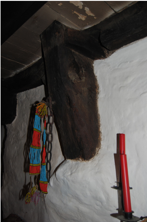
Plate 16: West foot of Cruck C2, note projecting
