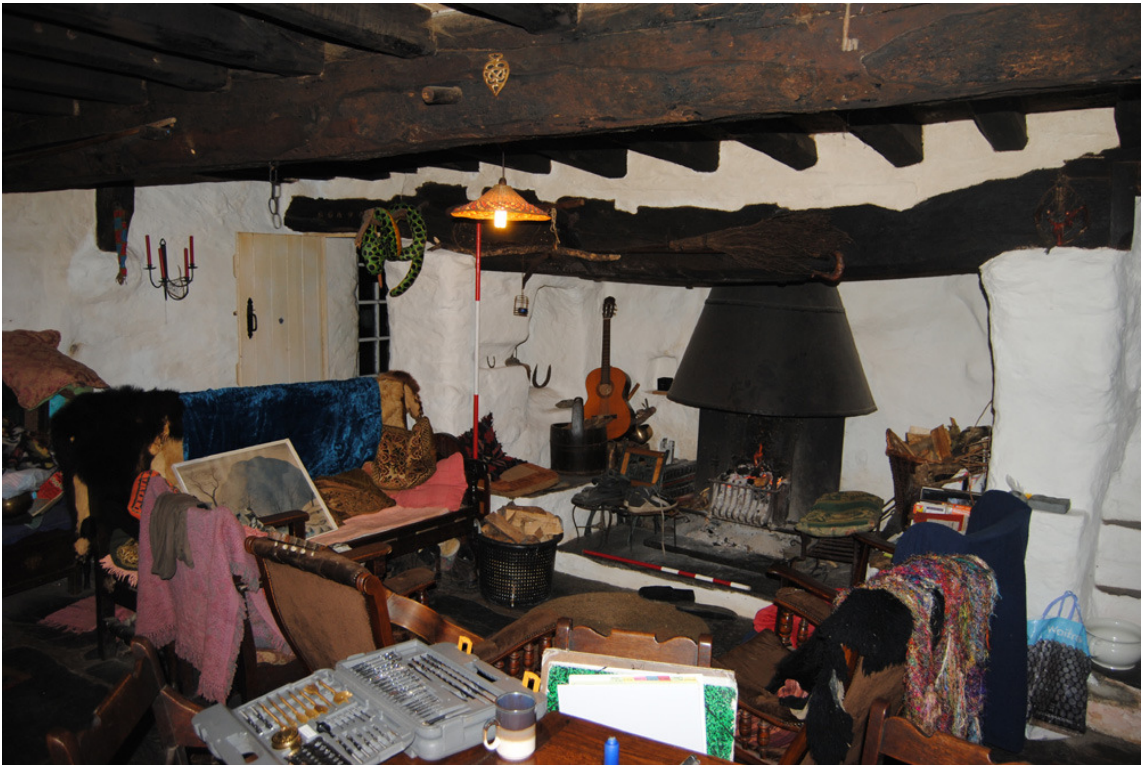
Plate 8: Room [GF01] looking south-east with inserted stack within Bay 3.
