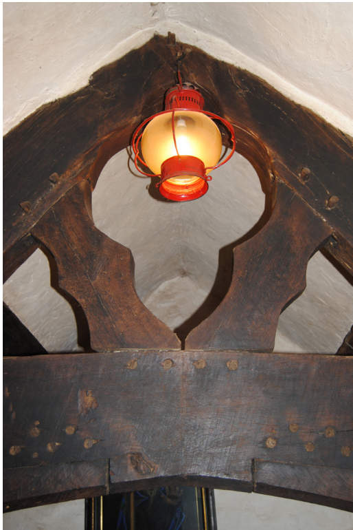
Plate 24: Cruck C2; cusping to v-struts.
