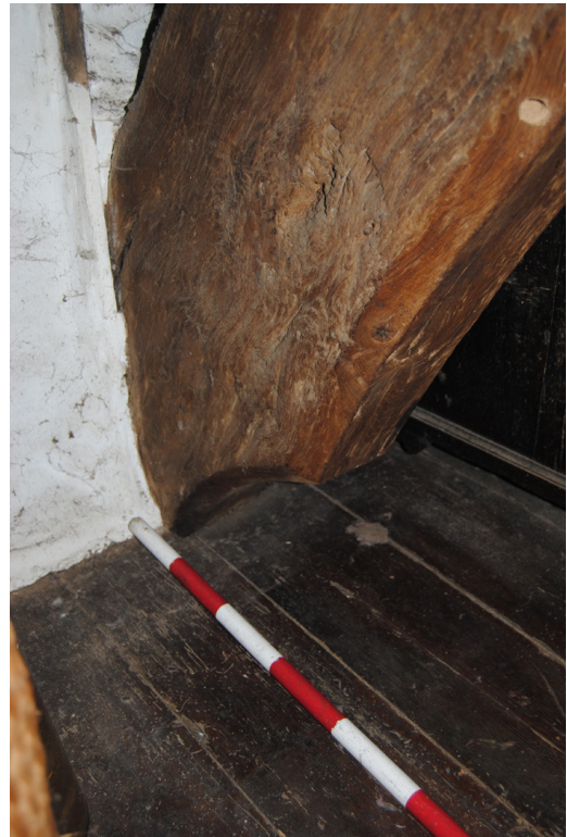
Plate 25: Cruck C2; cusping to western blade.
