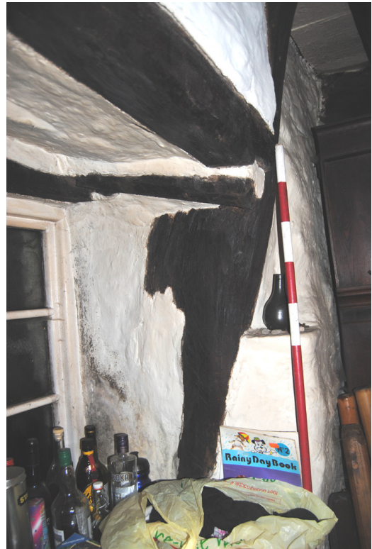
Plate 17: East foot of Cruck C2.
