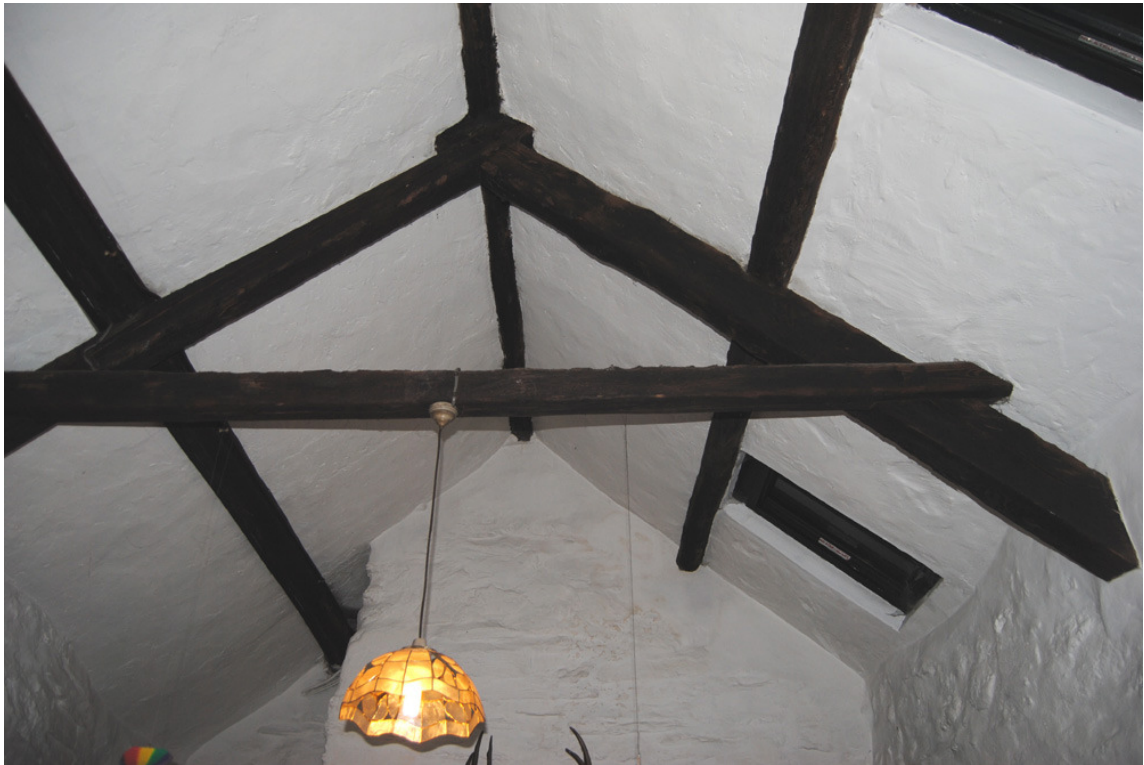
Plate 36: North-east extension roof structure.
