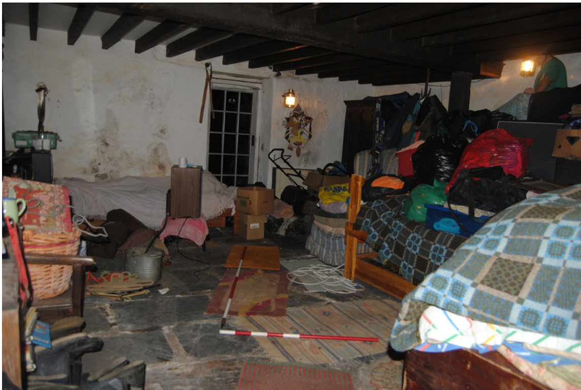
Plate 20: Room [GF06] (Bays 4/5) looking south-west.
