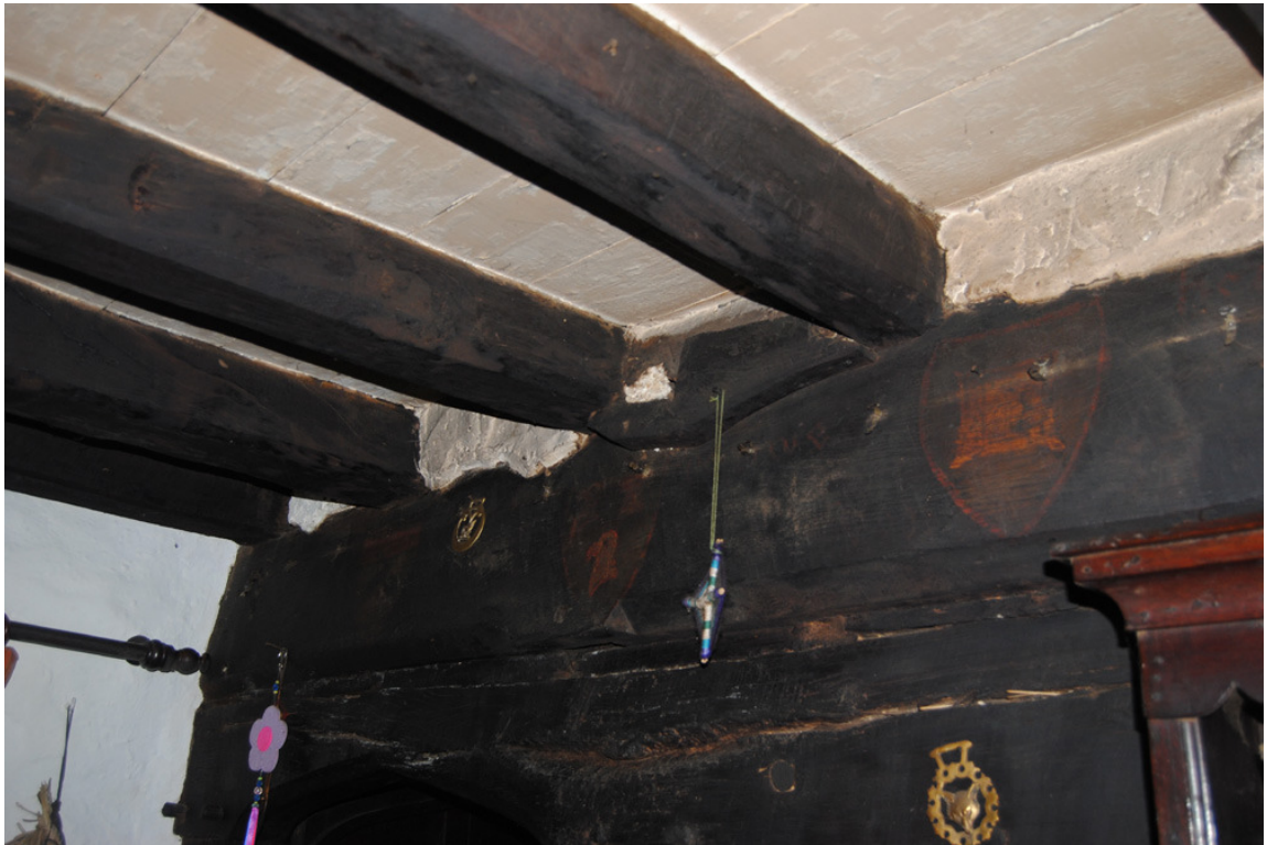
Plate 14: Joists of inserted floor rest upon tie of cruck C1 (NB: heraldic panels of c.1941)
