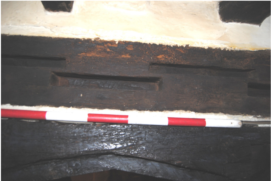
Plate 19: Staggered mortices for former 'post and panel' ceiling to north face of dais head-beam (= tie of C1).
