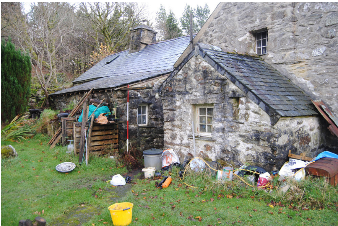
Plate 7: Single-storey extensions to north elevation of primary and north-east range.
