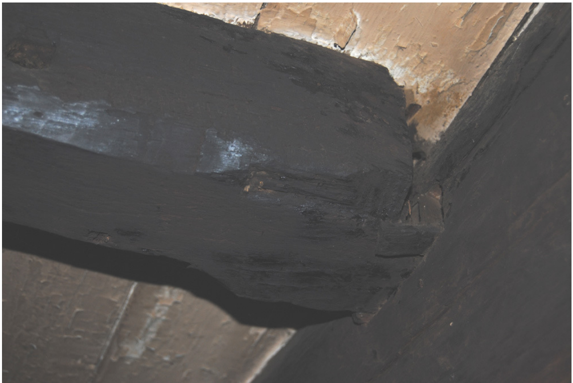
Plate 15: Common joist of inserted floor jointed to principal beam with bare-faced soffit tenon.
