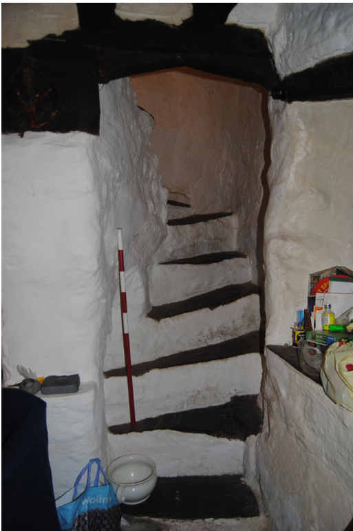
Plate 9: Winder stair to west of stack.
