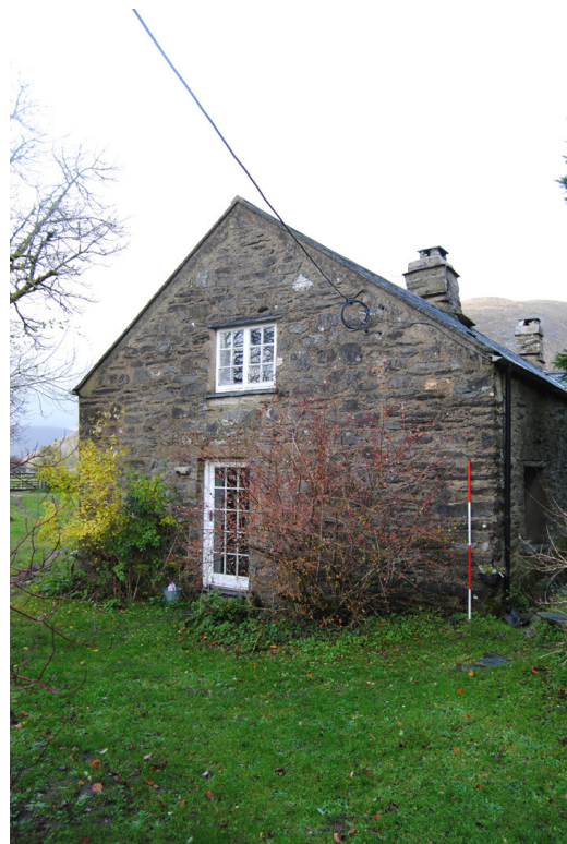
Plate 3: Primary range, south elevation.
