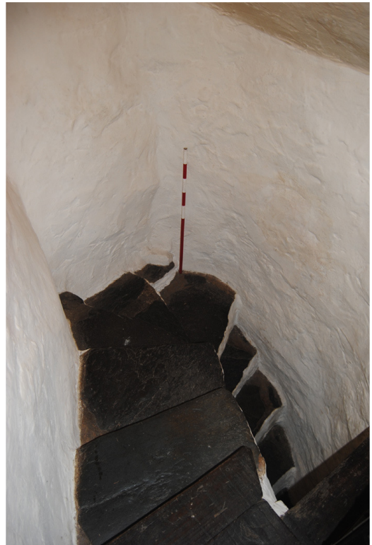
Plate 10: : Winder stair to west of stack (↓).
