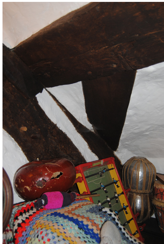
Plate 30: Surviving wind-brace at C3 (E).
