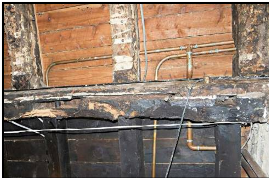
Figure 12: Ceiling beam over fireplace showing mortises in screen.
