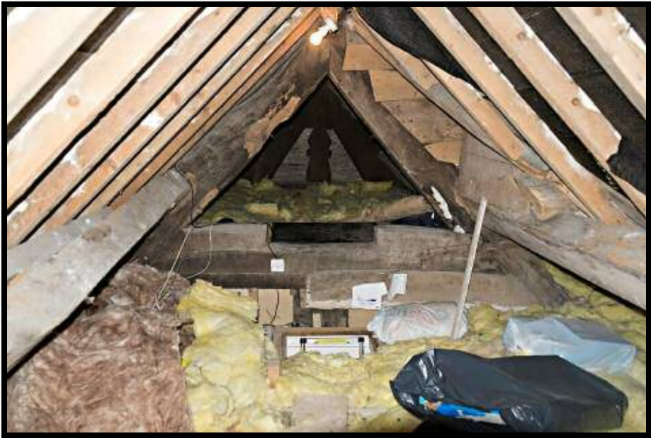
Figure 21: In Middle ground is Truss 2.
