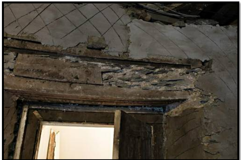
Figure 14: Re-used timber - rebated rails, holes and oddments.
