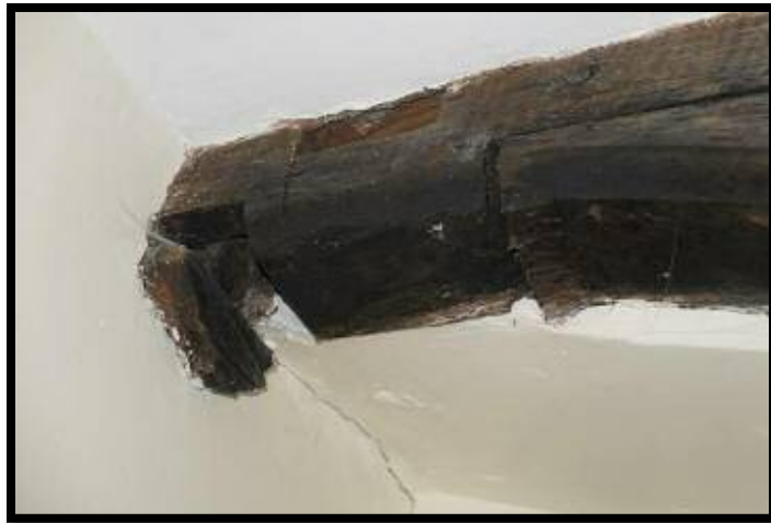
Figure 18: Bottom of principal with stud and mortise.
