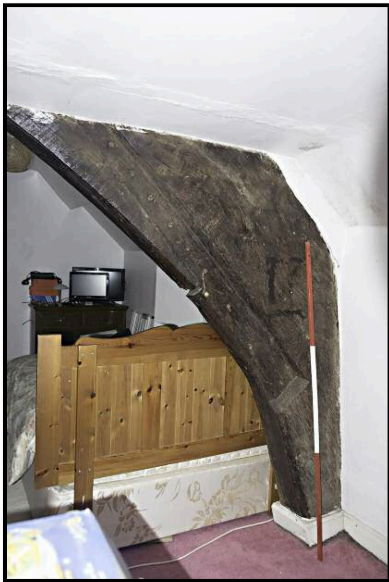
Figure 17: Left blade of cruck Truss 1. Additional decoration on 'rear' of arch braced cruck truss
