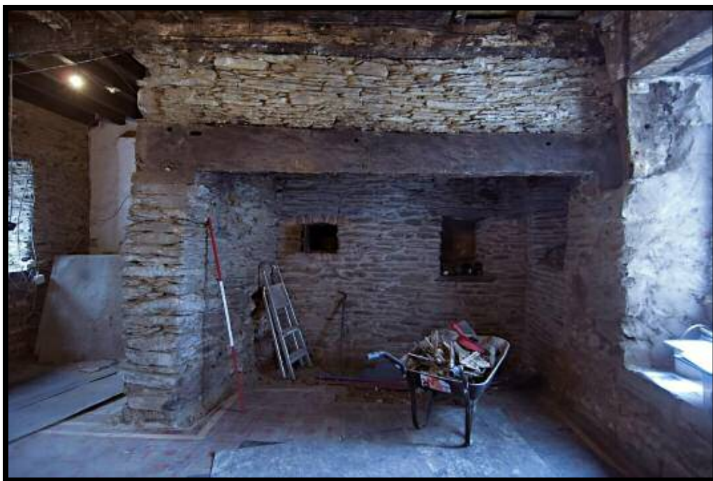
Figure 11: Inserted fireplace in hall.
