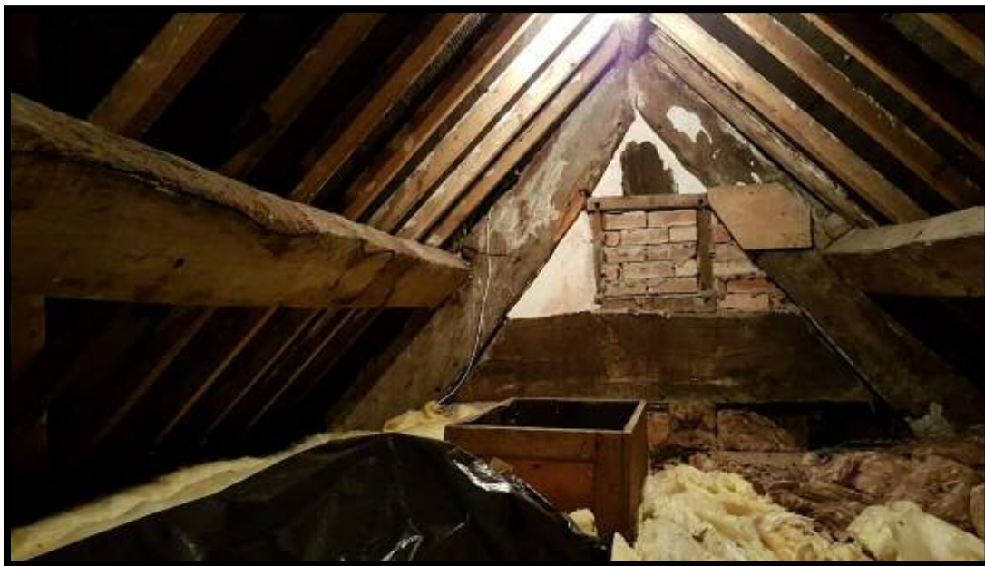
Figure 22: Truss 3. Central post at apex and several posts or studs drop from collar.
