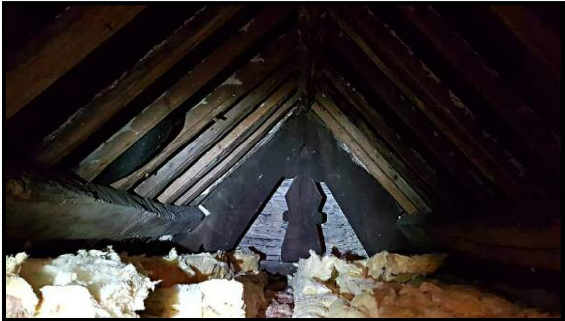
Figure 20: Unusual decorated king strut on Truss 1
