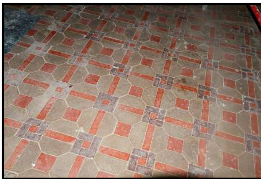
Figure 8: Ceramic tiled floor in hall.
