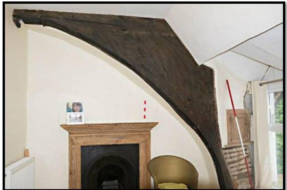
Figure 16: Right blade of Truss 1. Arch-braced.
