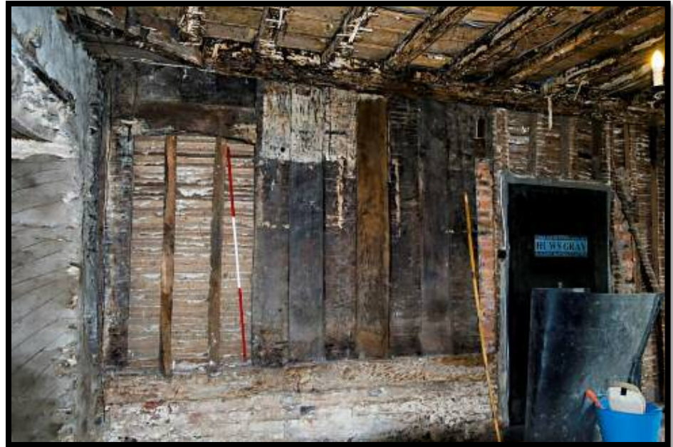
Figure 9: Remnant of plank & muntin screen.
