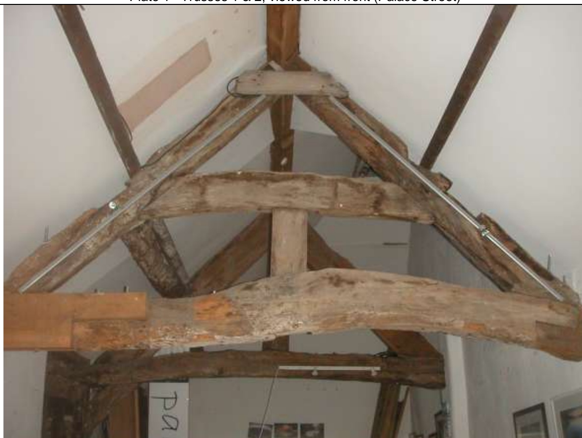
Plate 2 Trusses 2 & 3, viewed from rear
