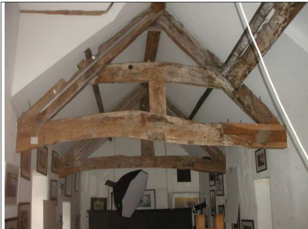
Plate 1 Trusses 1 & 2, viewed from front (Palace Street)
