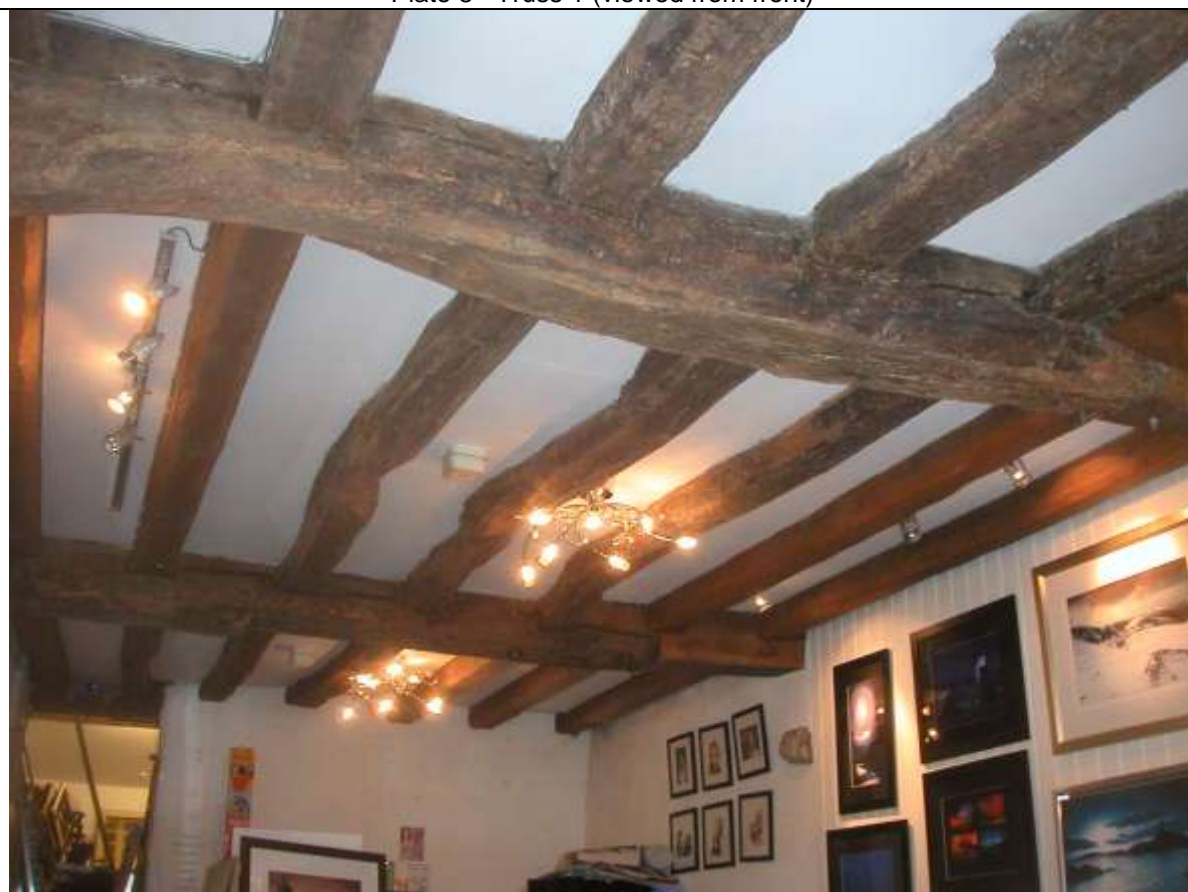
Plate 6 Ceiling to ground floor, beams below Trusses 1 & 2
