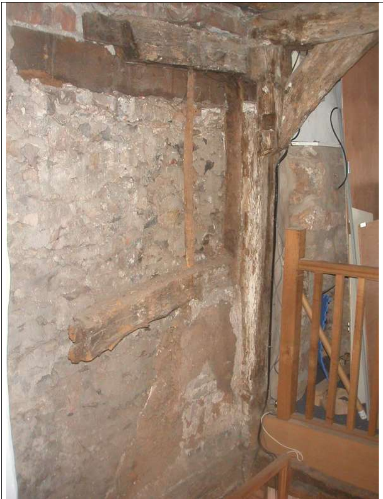
Plate 7 Oak framed wall on north side (with wattle & daub infill)
