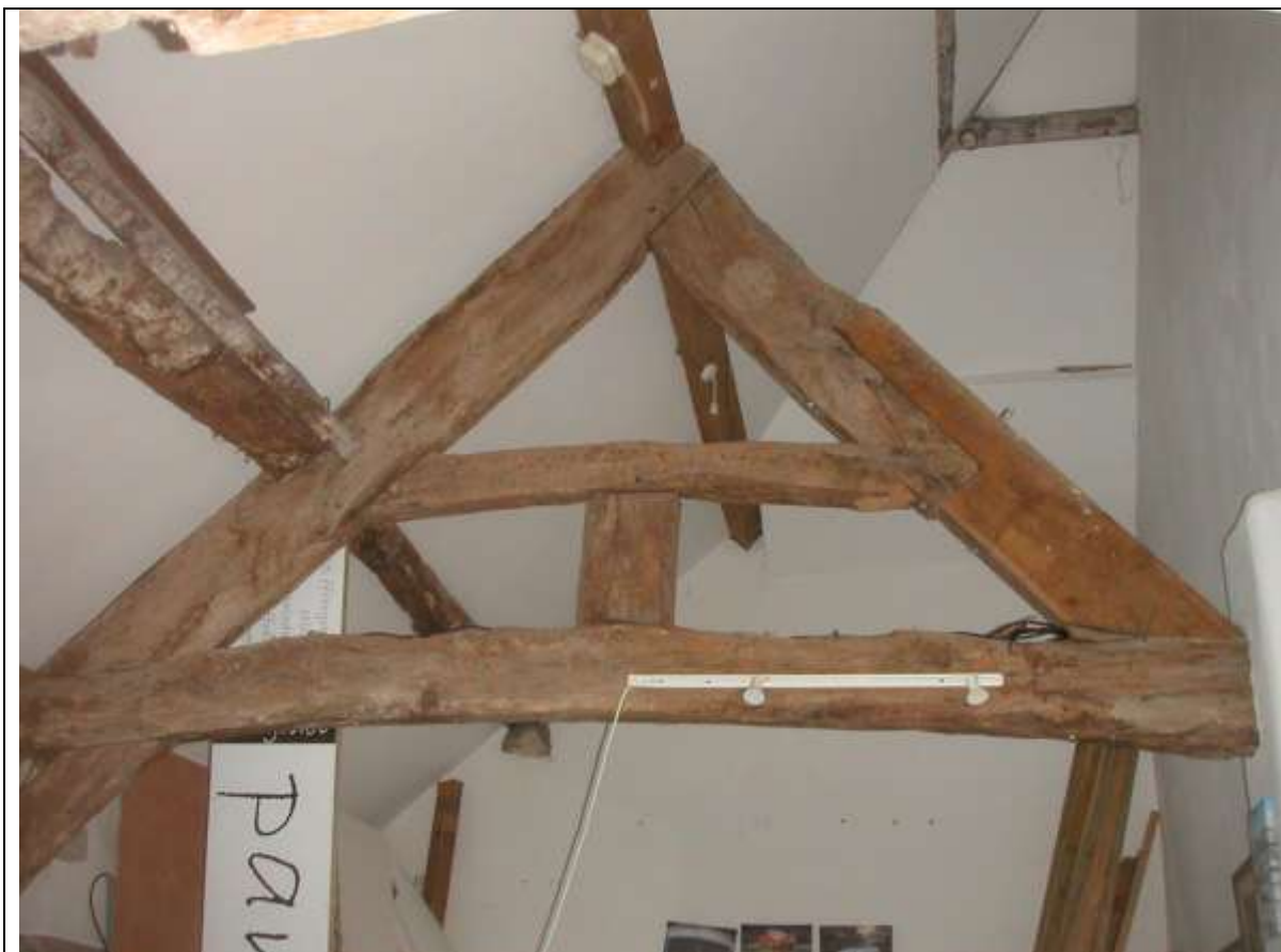
Plate 3 Truss 3 (viewed from rear)
