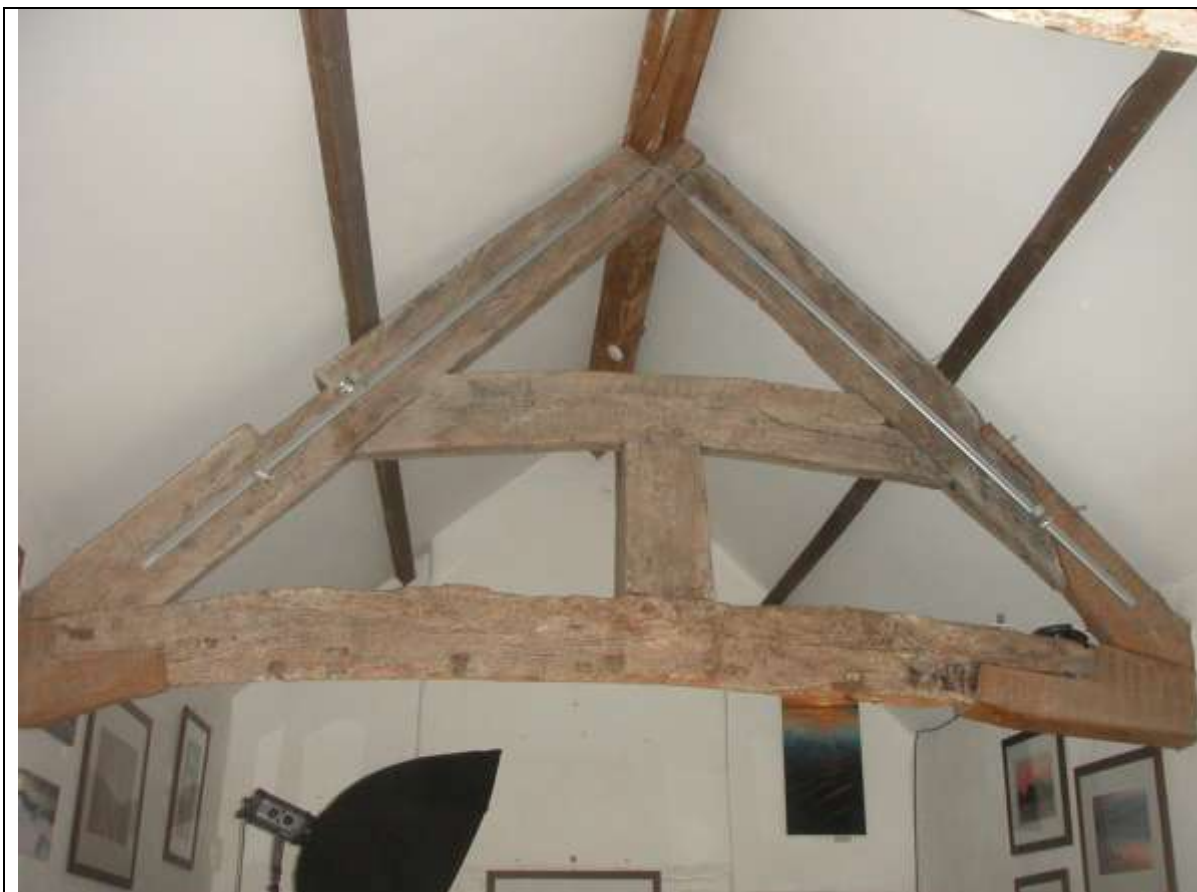
Plate 5 Truss 1 (viewed from front)
