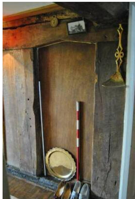
Plate 28: Primary doorway (blocked) within P&P partition [F1].
