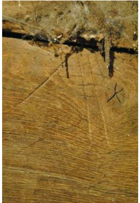
Plate 34: Scratched numerals; Truss T3 (wind-brace).
