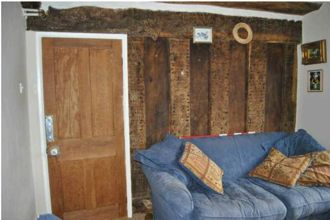
Plate 14: Post-and-panel partition to cross-passage, as exposed within [G4].
