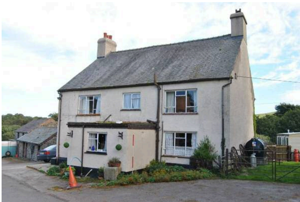
Plate 6: West (original rear) elevation, oblique view looking north-west with single-storey utility extension (post-1953; compare Figure 3b). Note general drop in ground level from south to north (left to right).
