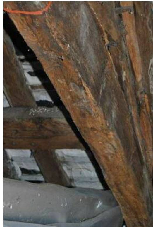
Plate 42: Secondary stave holes to soffit of arch-brace; Truss T11 .
