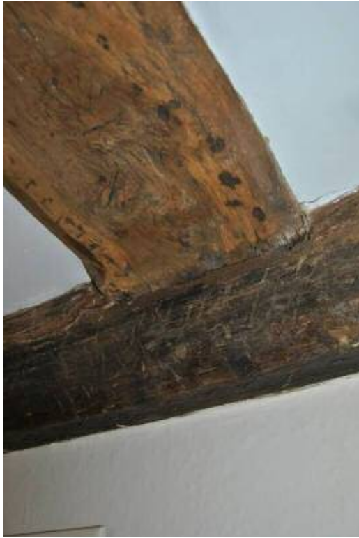
Plate 15: Detail of 1ft wide ceiling joist over [G4].
