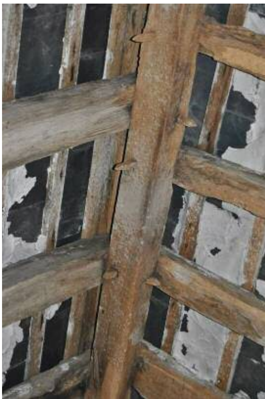
Plate 43: Ridge-piece over Bay III with pegs securing staggered primary common rafters.
