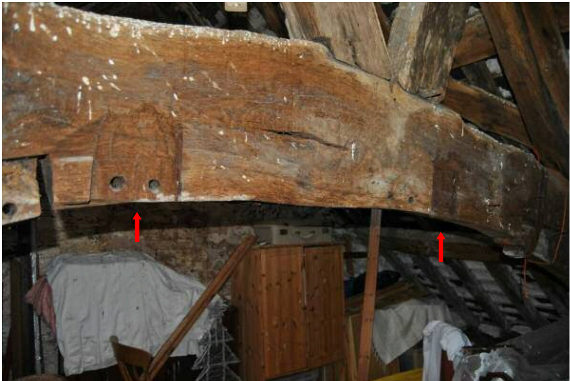
Plate 43: Pegging for secondary infill of truss T1.
