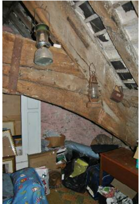
Plate 36 : Detail of arch-brace (Truss T3).
