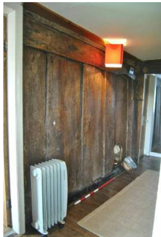
Plate 25: Post-and-panel partition at south side, [F1].
