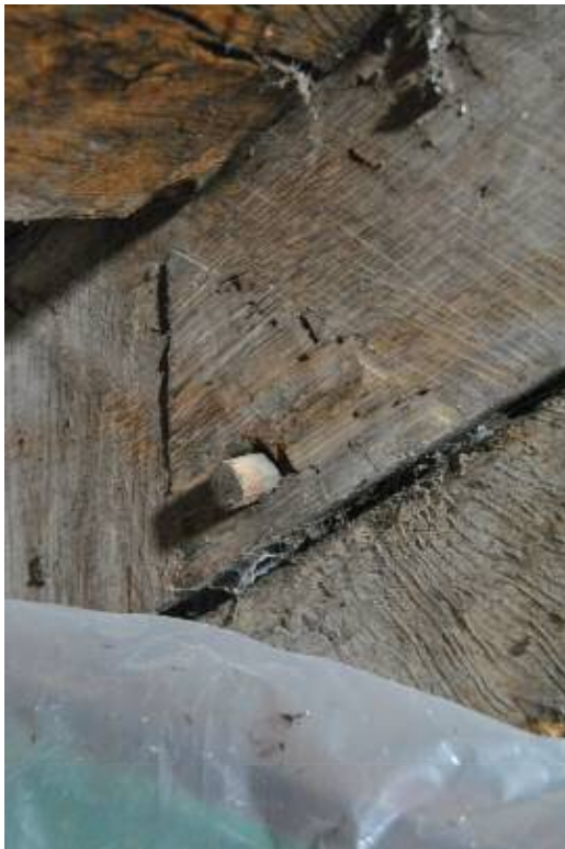
Plate 39: Distinctive evidence for trestle sawn timber; Truss T1 (west principal).
