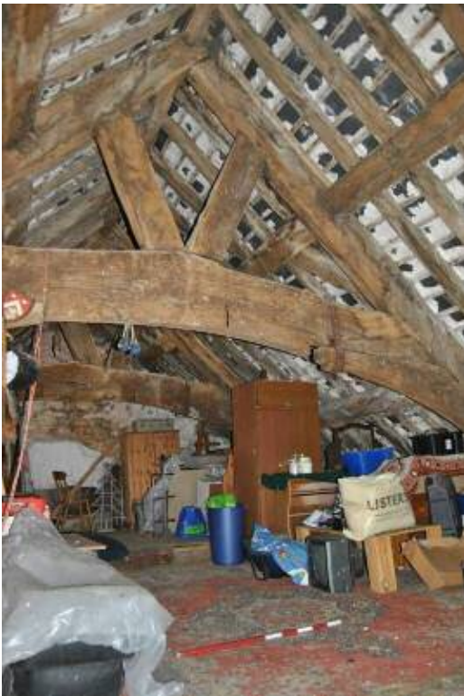
Plate 33: Roof-space looking south with Truss T2 to foreground.
