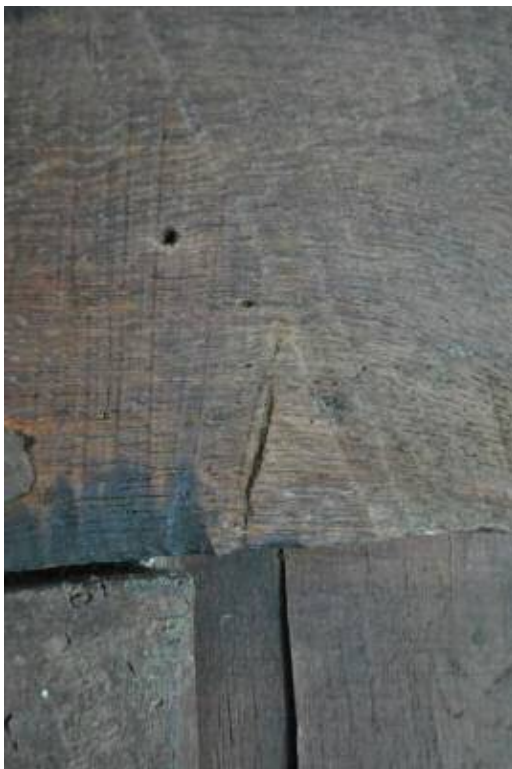
Plate 27: Evidence for trestle sawing in head beam of P&P partition.
