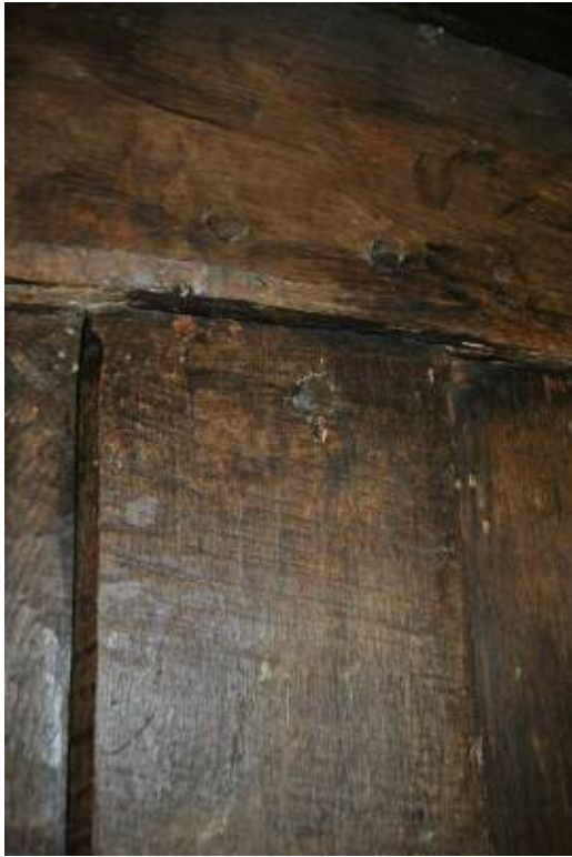
Plate 13: Joinery detail of post-and panel partition.
