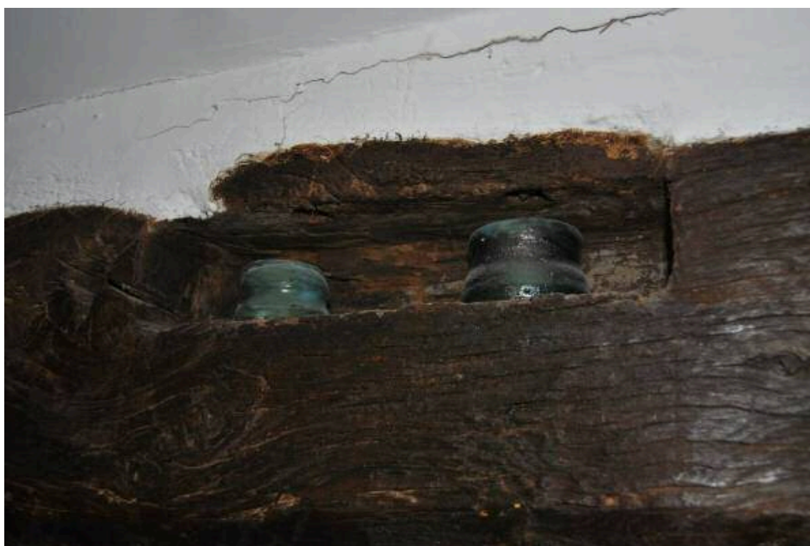
Plate 30: Detail of joist socket (NB. double peg-holes).
