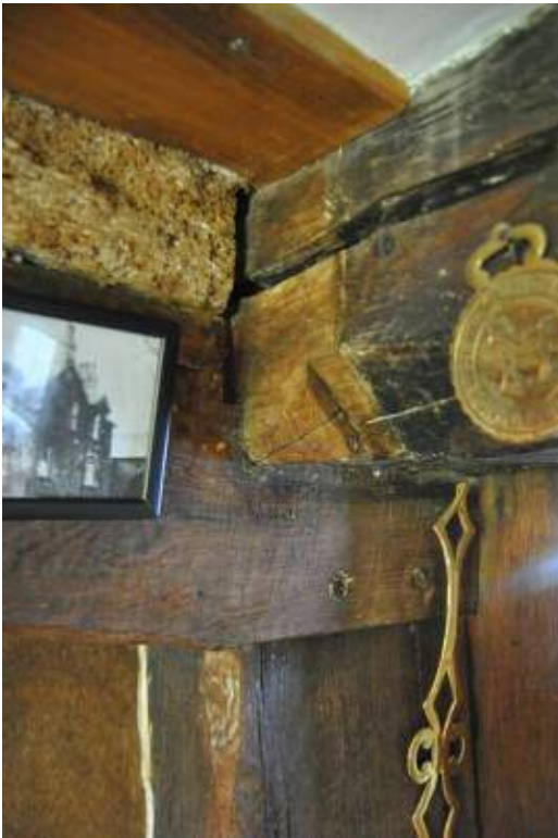
Plate 31: Stop-chamfered spine beam at P&P partition.
