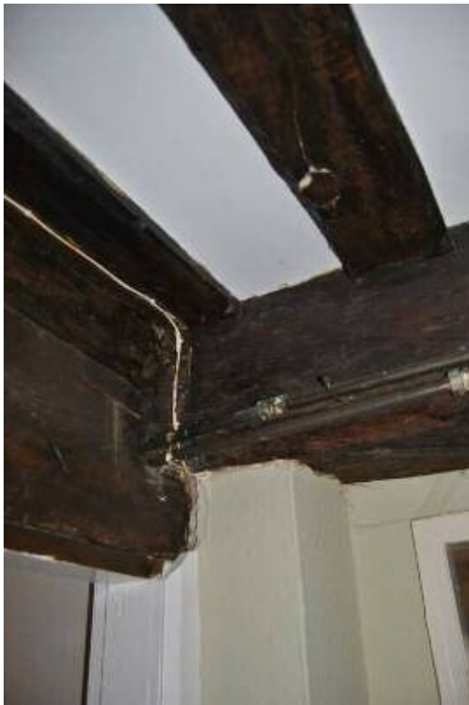
Plate 19: South end of spine beam at P&P partition [G1a].
