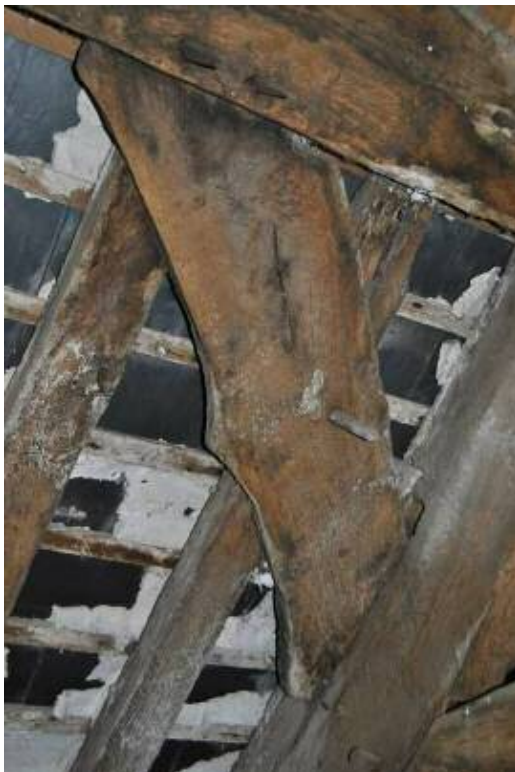
Plate 41: Detail of cusped wind-bracing.
