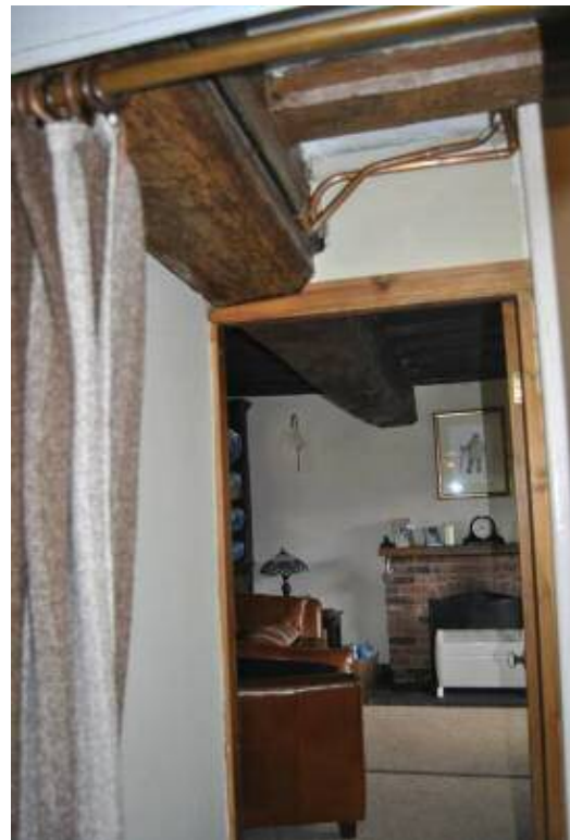
Plate 18: Axial 'spine-beam' extending across [G1b] and [G2].
