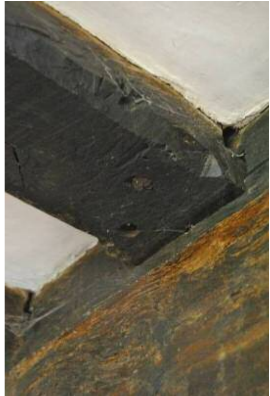
Plate 20: 7in., stop-chamfered common joist over [G2].
