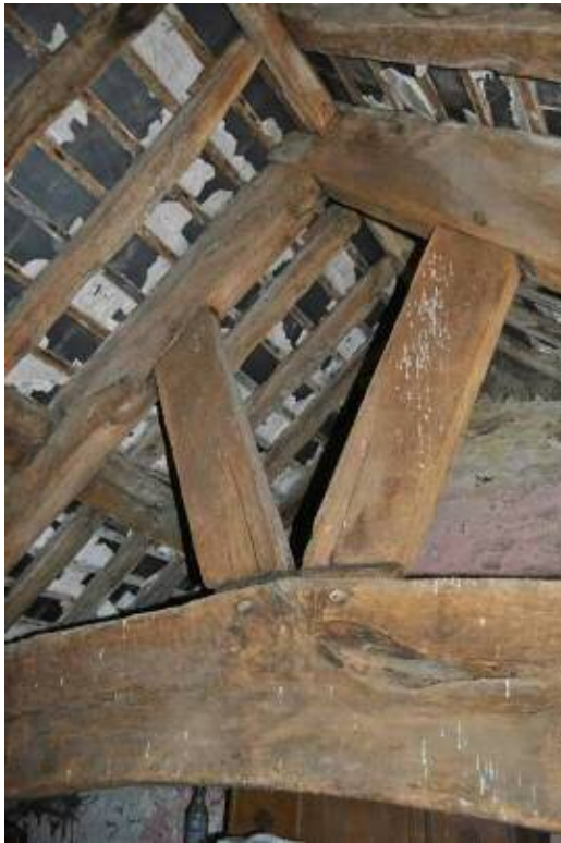
Plate 35: Detail of v-strutting above cranked collar (T3).
