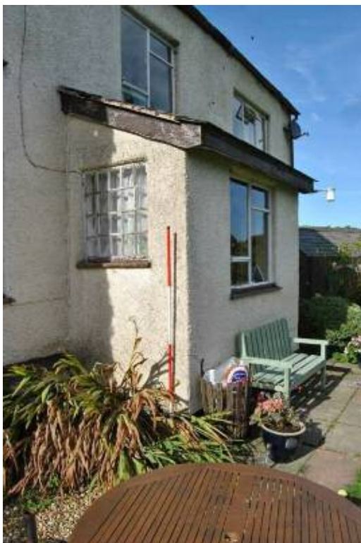
Plate 4: Pent-roofed porch appended to east elevation after 1953.
