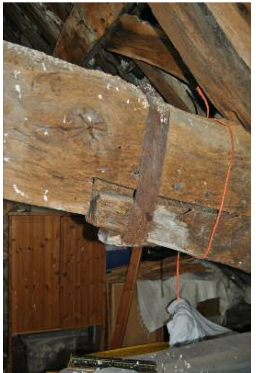
Plate 38: Repair of arch-brace/collar joint with iron strap and wedge.
