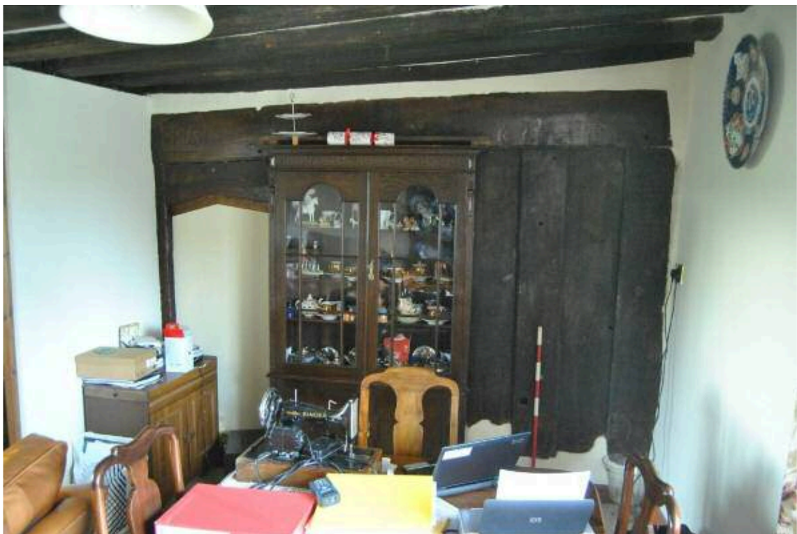
Plate 21: Post-and-panel partition to south side of [G2] (assumed relocated from cross-passage).
