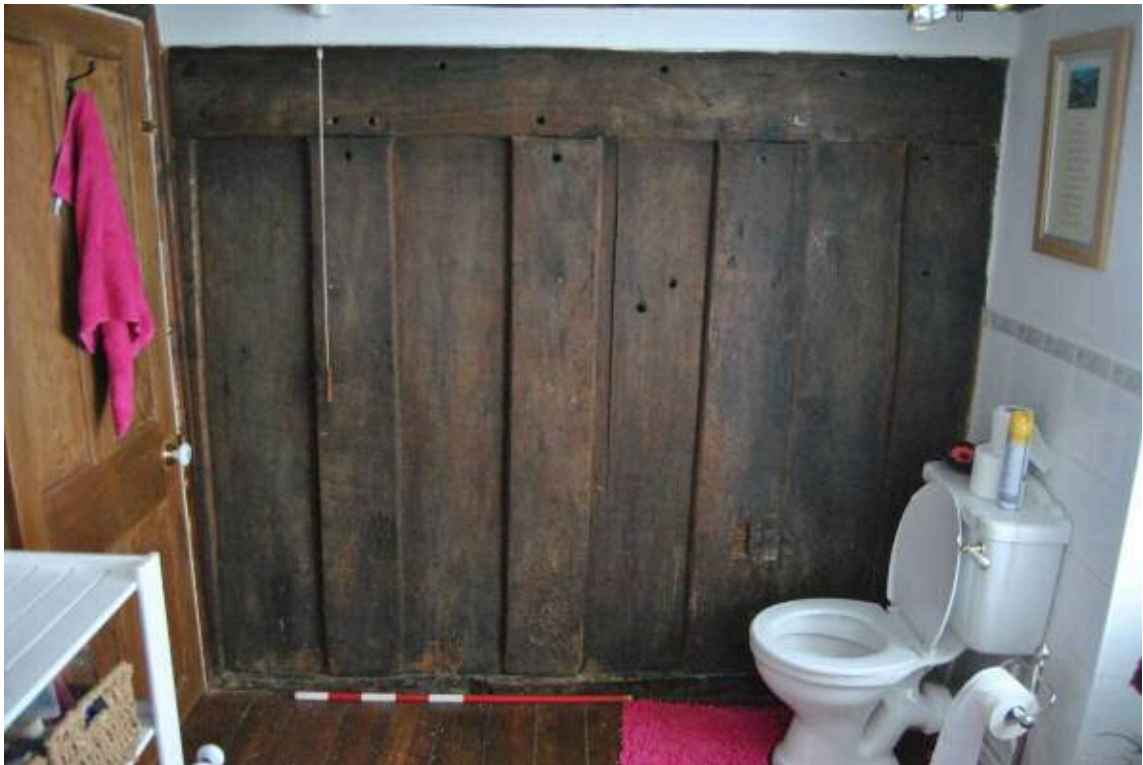
Plate 26: Continuation of P&P partition, exposed within bathroom [F4].
