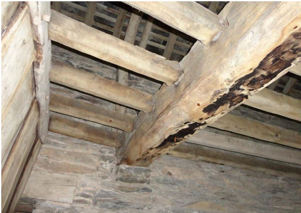
Figure 3. Photograph showing the locations of fedw1 (main beam) and fedw3 (joist)
