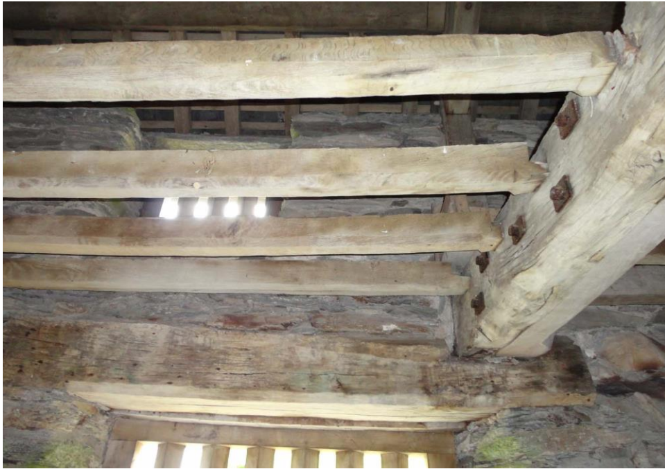
Figure 5. Photograph showing the location of samples fedw6 and fedw7 (joists)
