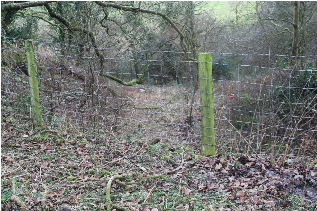
Photo 17: Facing south. Dry water channel heading south-southeast from the east side of Castell Pen-yr-Allt, possibly once joined with the northeast ditch, which contained water.
