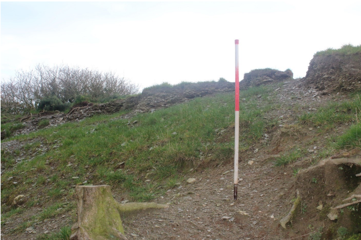
Photo 16: Facing south. Close up of erosion on the outside of the top of the bank on northeast side of Castell Pen-yr-Allt, with a 1m scale.
