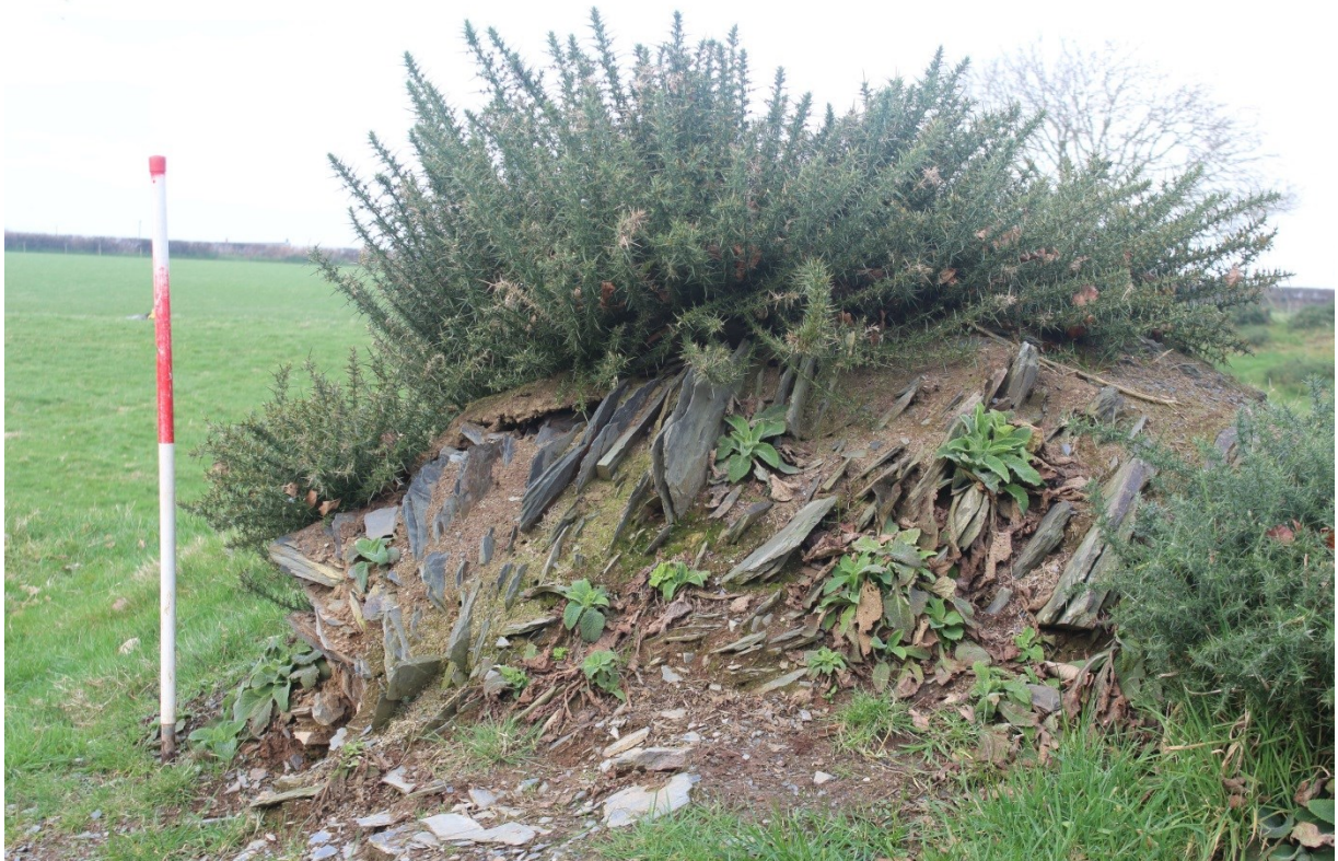
Photo 5: Facing north. Stonework remains on top of the motte at Castell Pen-yr-Allt, with a 1m scale.
