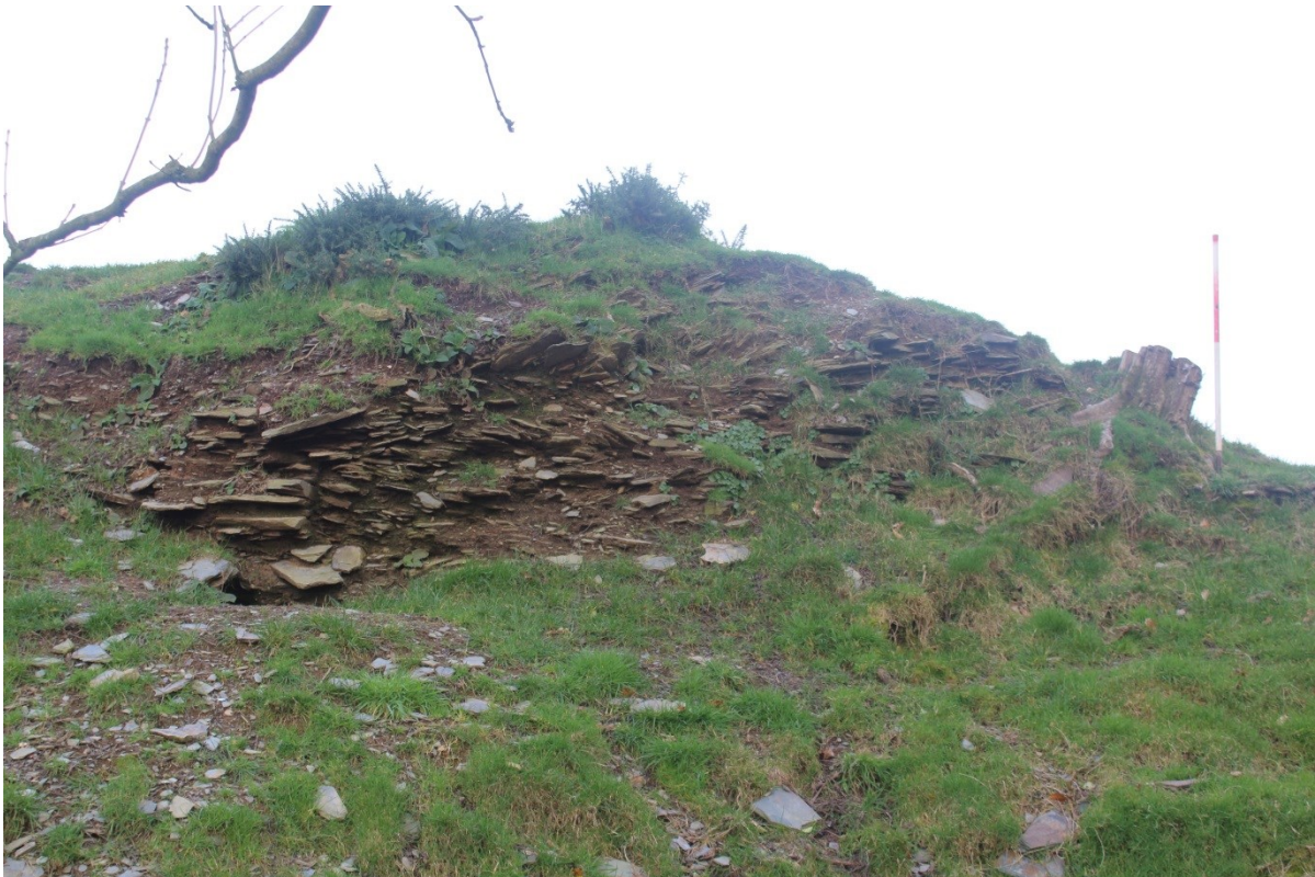
Photo 10: Facing northeast. Part of the remains of a bank and/or stone building on the west side of Castell Pen-yr-Allt, with a 1m scale.
