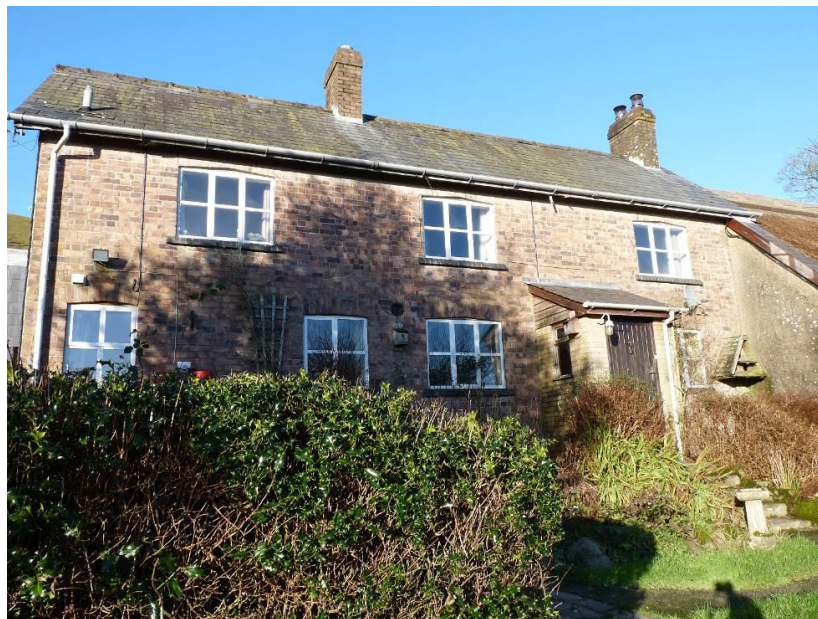
Fig.10: adjoining warden's cottage built in 1878
