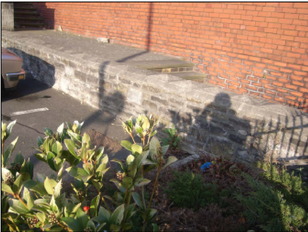
Plate 2 Possible surviving footing of north wall of Guardians Offices. View to north-west
