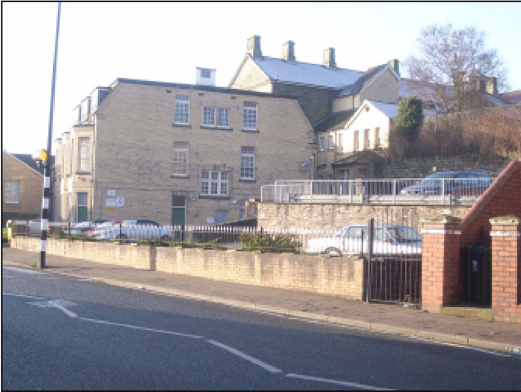
Plate 1 Foreground, former site of Board of Guardians' Offices, Queen's Hill, now a car park; background, original block with modern flat roof and dormers, to rear of Queen's Chambers. View to south-west
