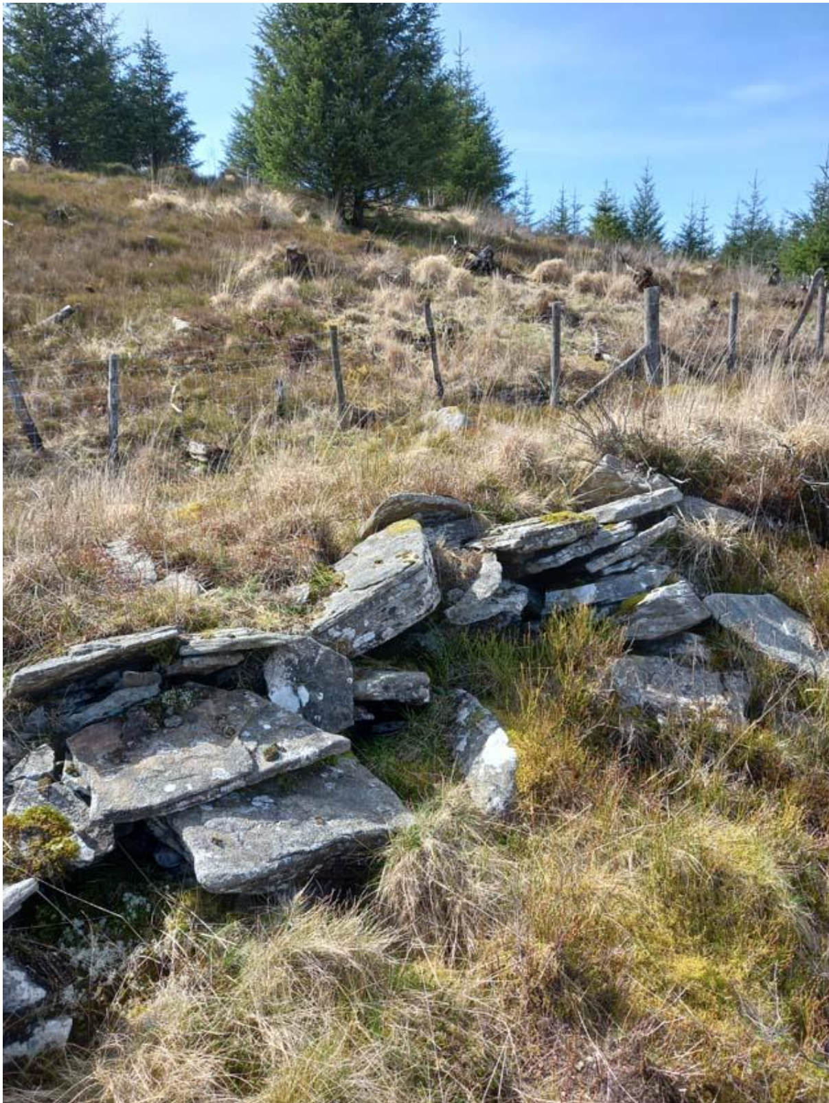
Figure 1 Ffos Toncenglau Dyke construction: horizontally laid coarse stone slabs (CPAT photo 5047-010)
