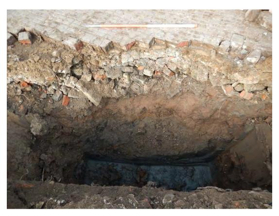
Photo 3: West facing section of the drainage trench excavation, showing the lower natural deposits (021) and (020), overlain by modern deposits (003), (002) and (001). 1m scale.
