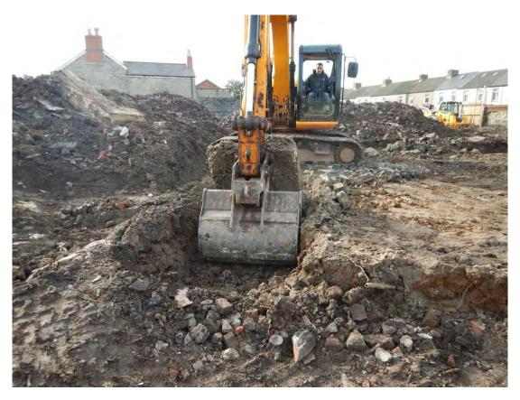
Photo 9: Concrete foundation of wall {009/016} during removal, looking north.
