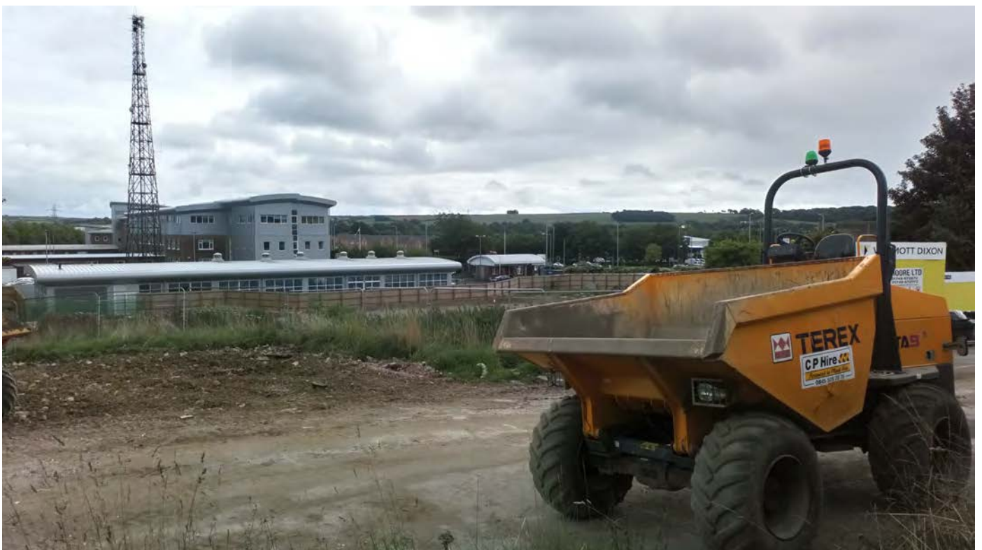
Plate 2: View south-east over the development site.
