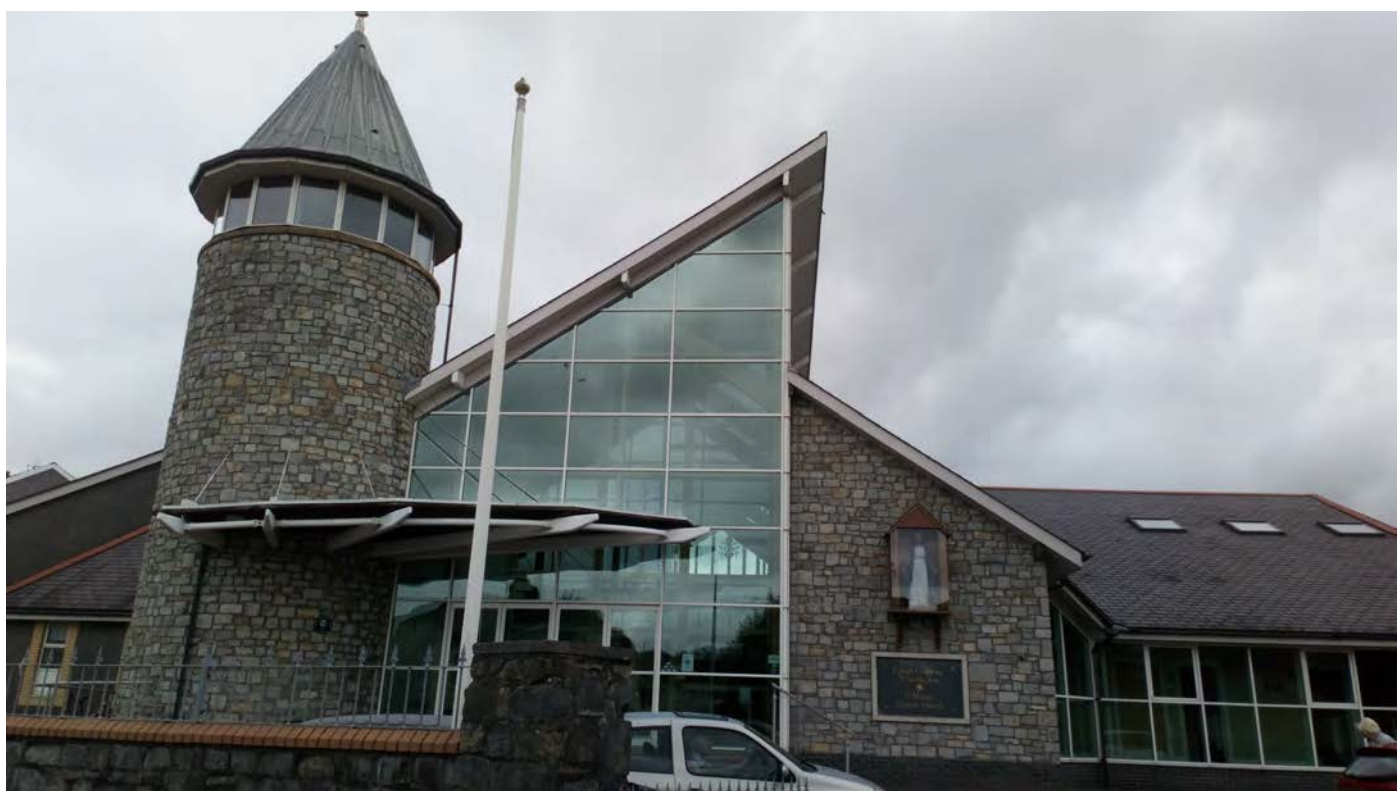
Plate 10: St Mary's Catholic Church (NPRN 13795).
