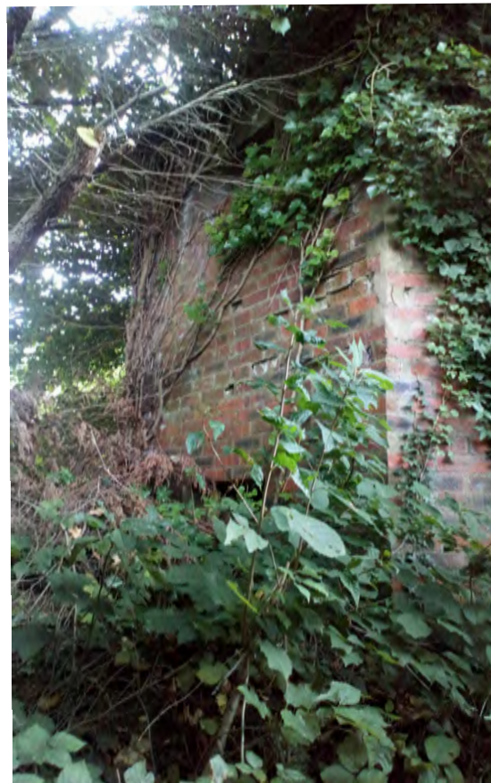
Plate 6: View north-east of the only exposed section of the pillbox (GM 605).
