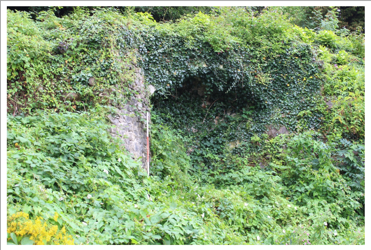
Plate 3: Close-up of arch, view from west
