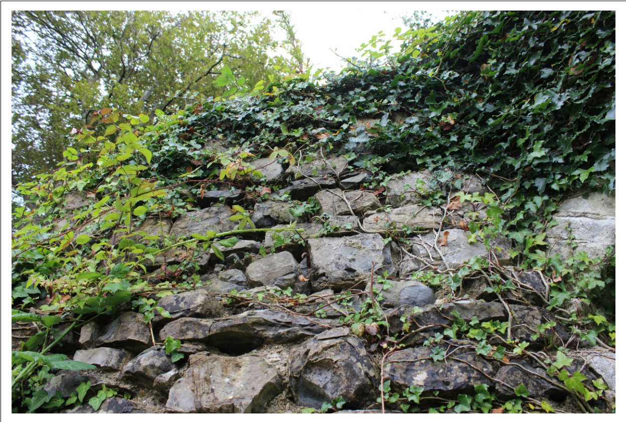
Plate 9: Close-up of northern retaining wall, view from west
