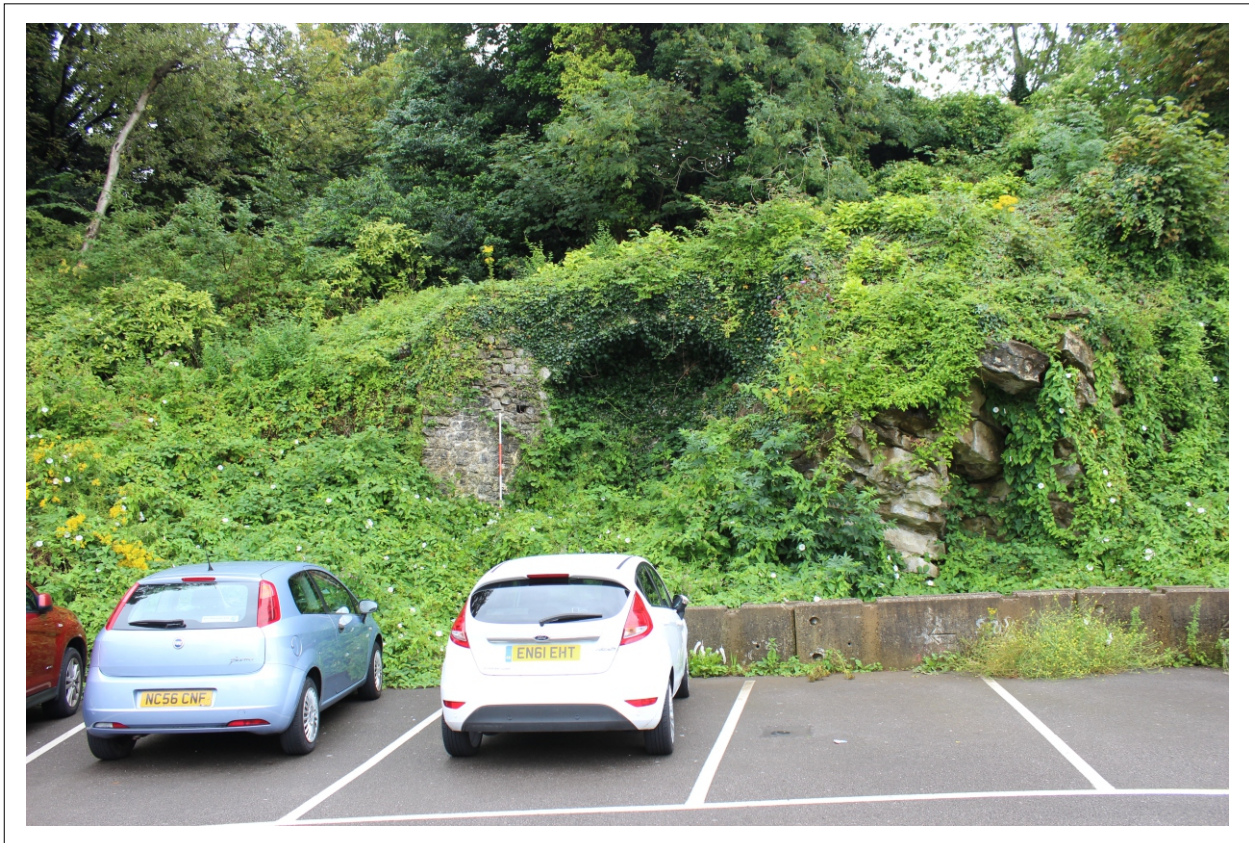
Plate 1: Western elevation, view from west
