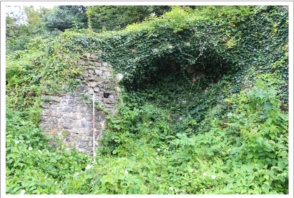
Plate 2: Western elevation, view from west
