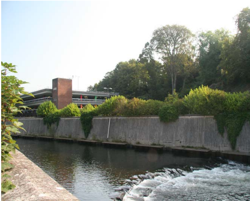
Rear of the multi-storey car park (southern end) seen from the western side of the Ogwr river (looking north-east)
