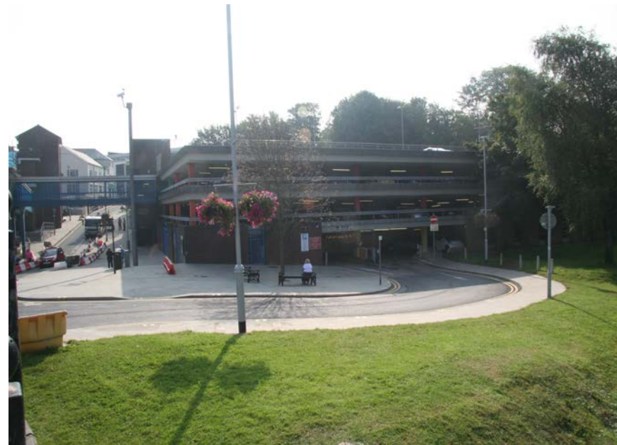
Multi-storey car park at bottom (western end) of the Rhiw (looking east)
